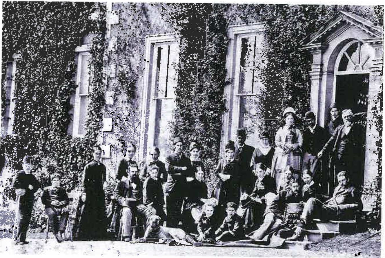
Fig 03: Photograph of James Garnett (seated off centre left) with other Garnett family members c. 1880's. It should also be noted that the door, stone surround in question is also present within this particular photograph. It also shows the steps differing to the steps which exist today which are likely to be replacements.
