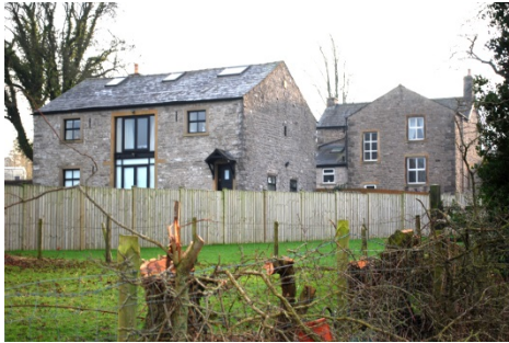
Mill Hey Barn has new larger openings formed
