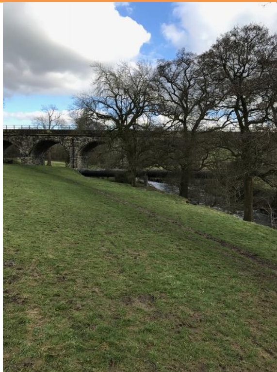
PLATE 5 – RAILWAY VIADUCT AND PIPE CROSSING ADJACENT TO SOUTHEAST BOUNDARY
