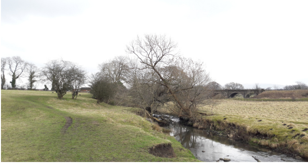
View of G32 facing east.
