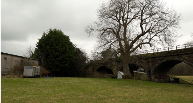
T30 in foreground. G28 and G29 in background.
