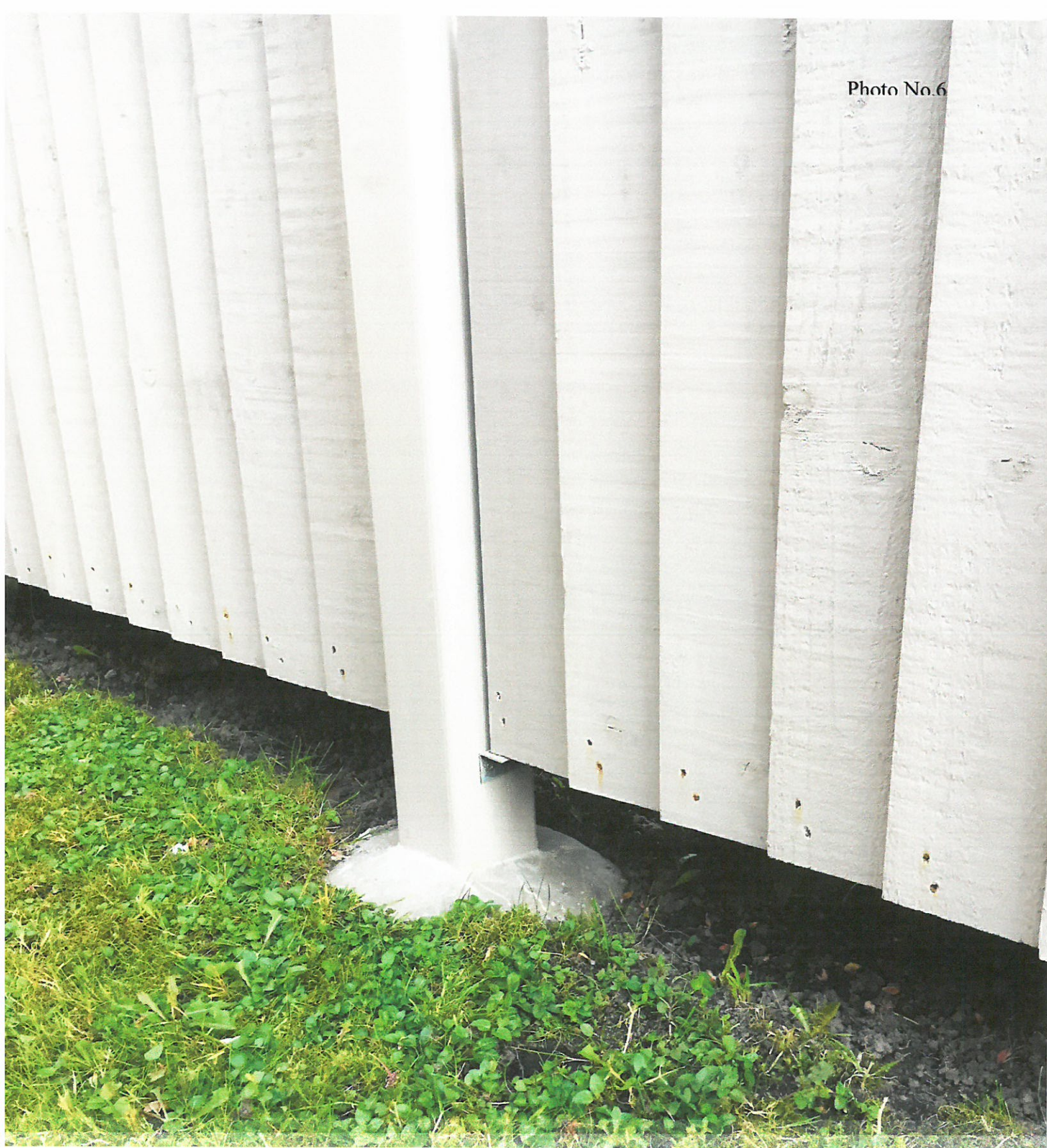
View from inside showing approx 300mm round hole with wooden fence post set in sloping concrete and 30 x 30 x 50mm galvanized angled piece screwed to fence post to support wooden fence panels from below (2 No. to each panel).
