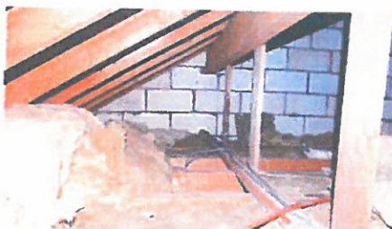
Figure 4: new roof void
