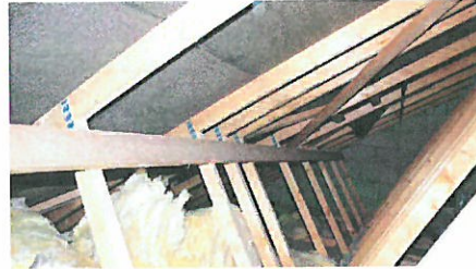
Figure 4: main roof void
