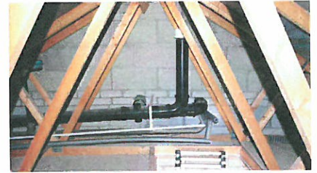
Figure 5: garage roof void
