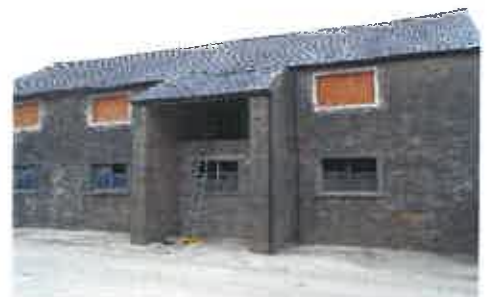
Figure 3: Barn 'B' front elevation
