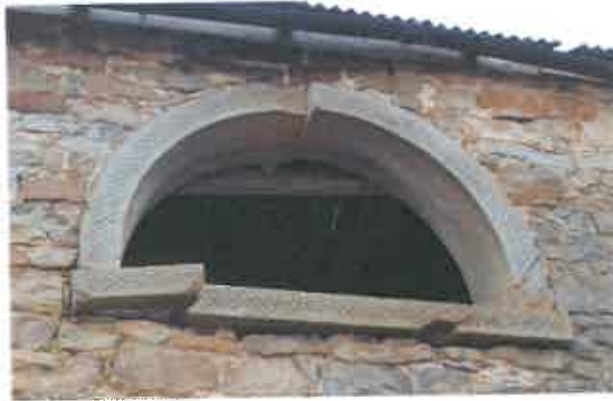
Photograph (16) – Illustrating the condition of the Storage Area window surround that needs replacing.
