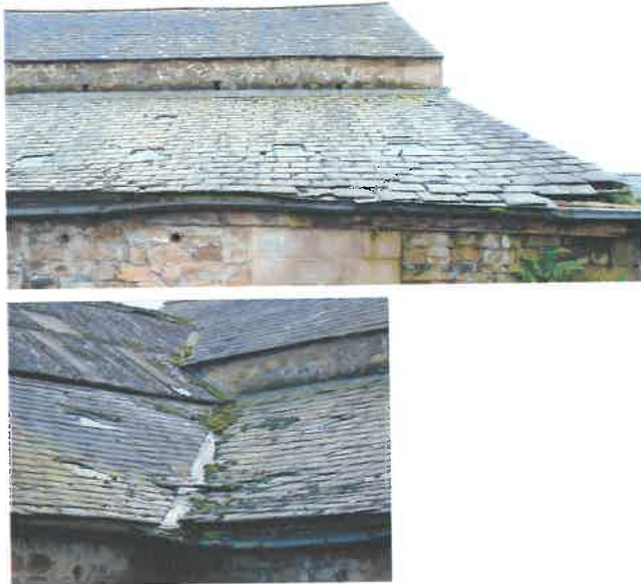
Photographs (8 and 9) – General condition of the lean-to roof.
