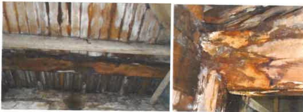
Photographs (6 and 7) – General condition of the lean-to roof.
