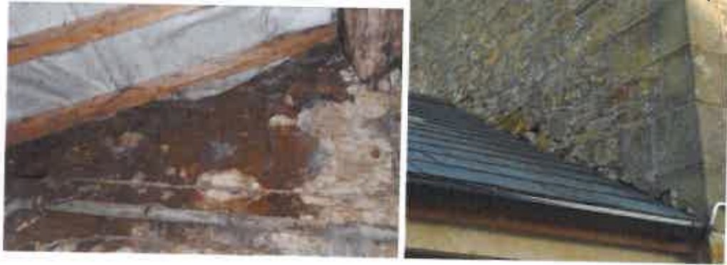
Photographs (10 and 11) – General condition of single storey roof.
