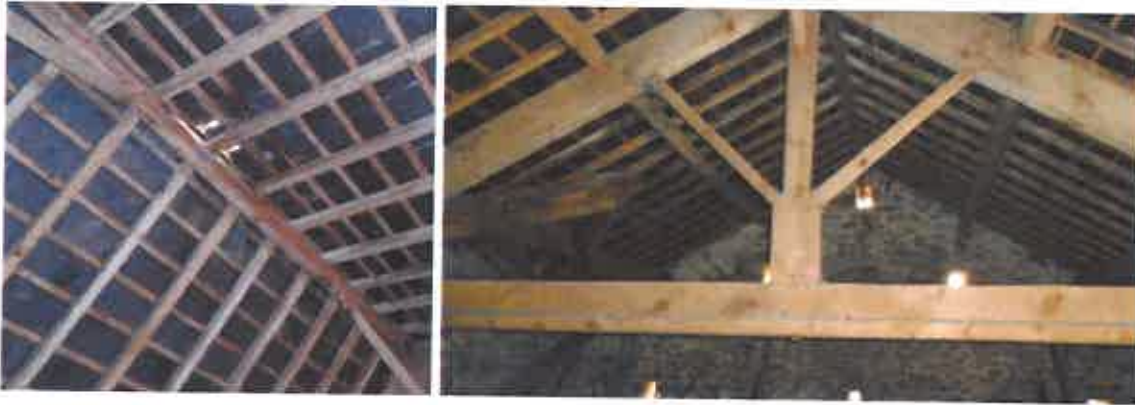
Photographs (1 and 2) – Roof structure to South West Barn.
