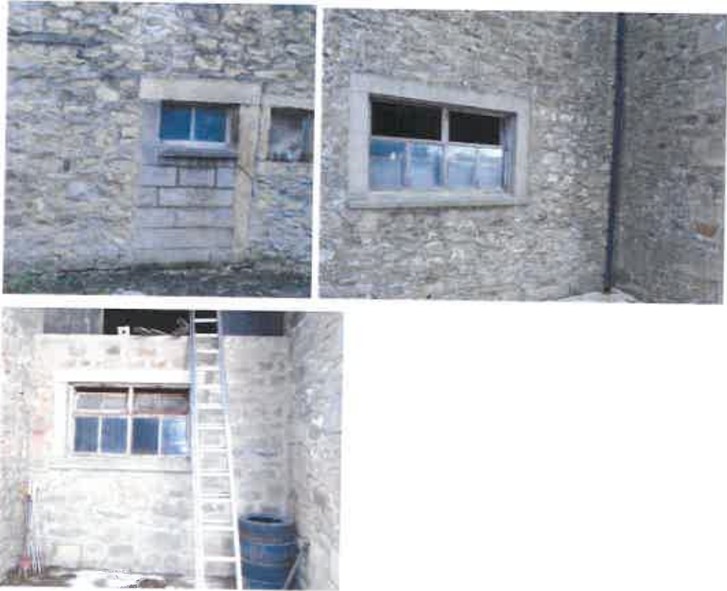
Photographs (17 - 23) – Illustrating the general condition of the walls.
