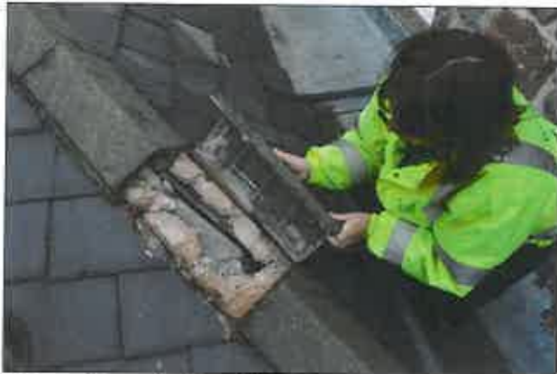
Inspection of ridge tiles
