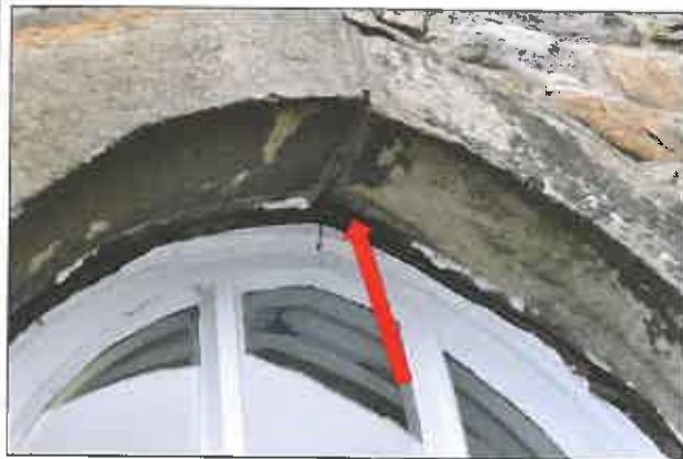
Smaller window on south west elevation – cavity marked with arrow
