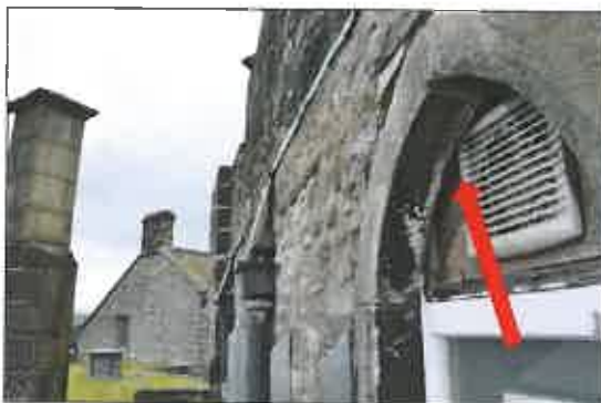
Larger window on south west elevation (roof access point) – cavities marked with arrows
