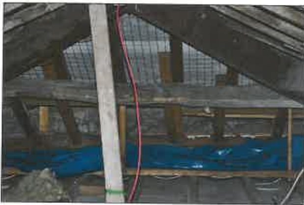
Roof void – north section
