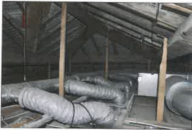
Roof void – south section
