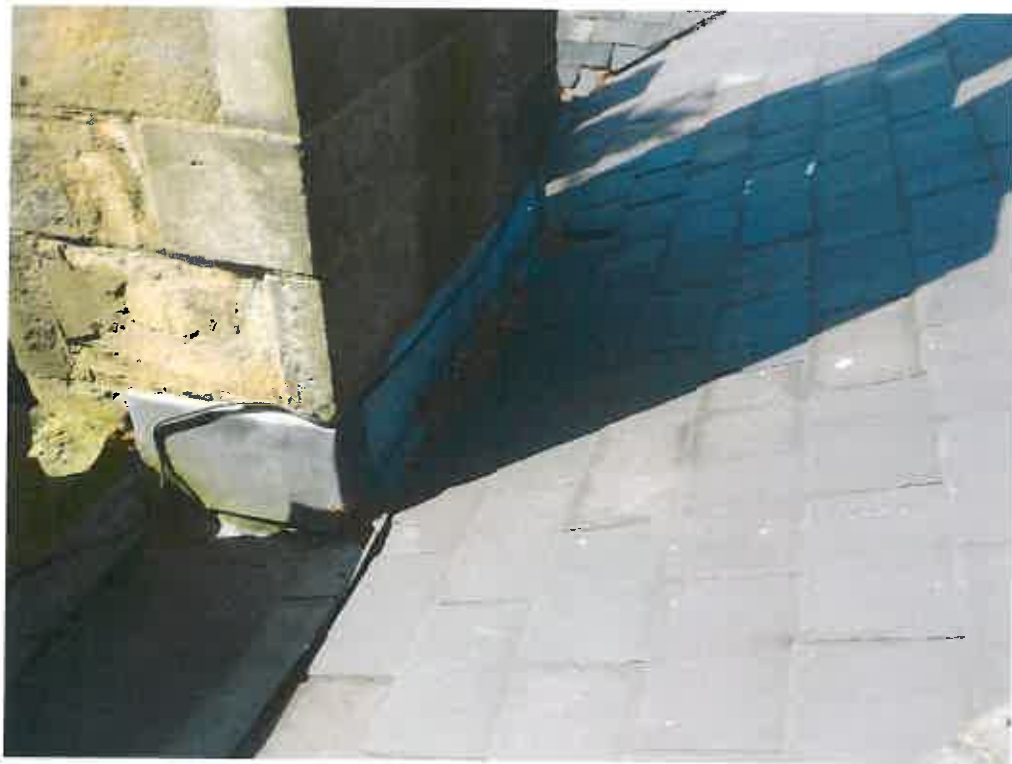
Figure 1 – shows highest part of the slate. To the sides of the chimney the slates would be in 5 or 6 tiers
