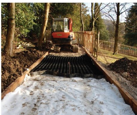
Fallbarrow Park, Windermere: CellWeb TRP® Installation
