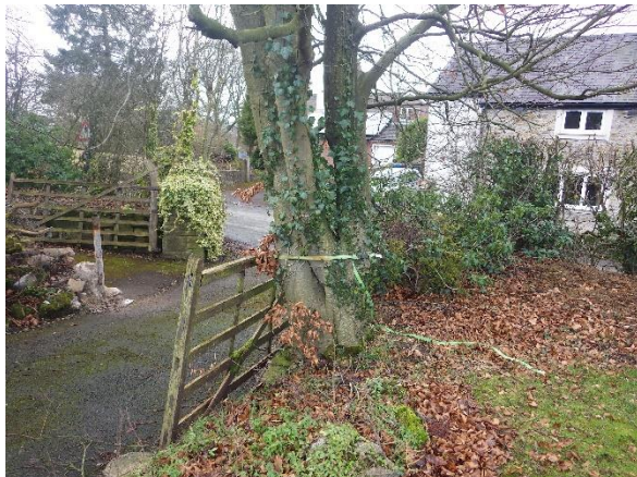
Figure 1: Tree T1 sitting atop a retaining wall, which will require demolition in order to construct driveway alterations as proposed
