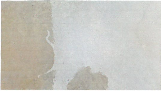
Power floated and Sealed concrete
