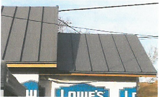
Standing Seam Roof and Cladding on Garden Room RAL7016— Example
