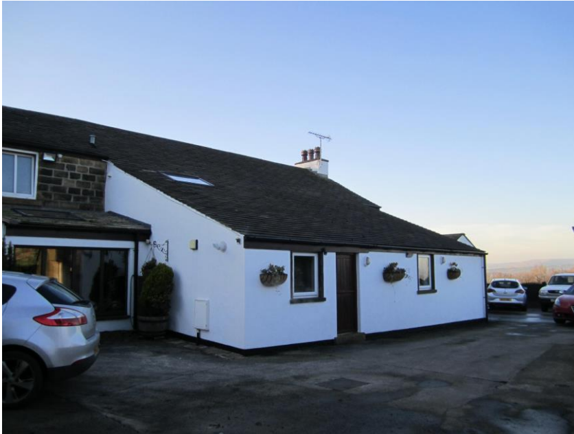
3 Front elevation of former barn.
