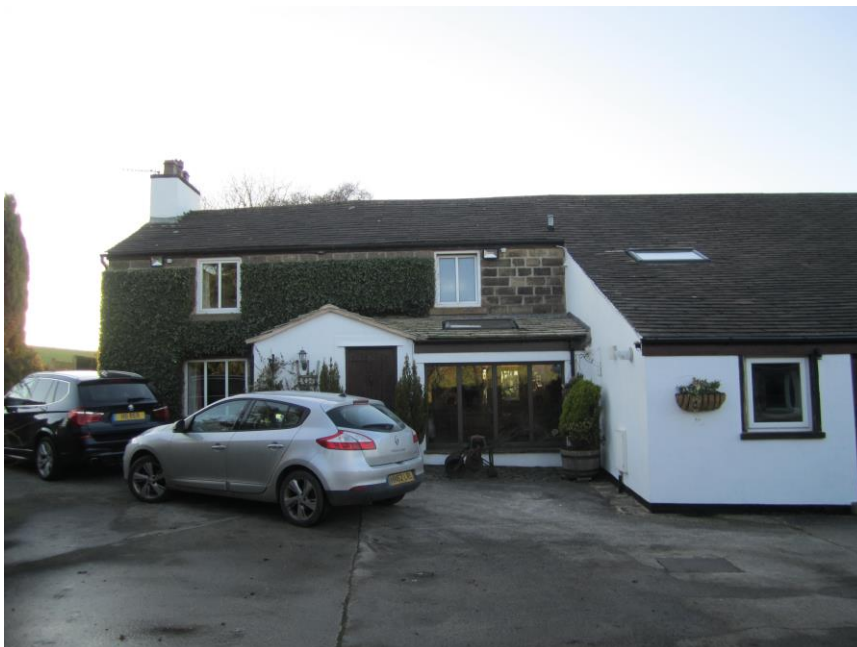
2 Front elevation of former farmhouse is stone
