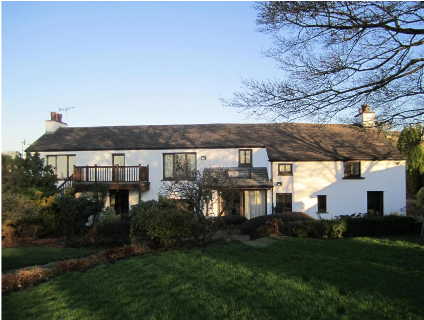
1 Rear elevation of former farmhouse and barn.
