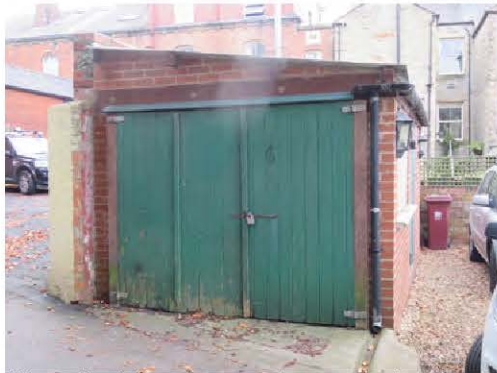
View of existing Garage, from rear alley.
