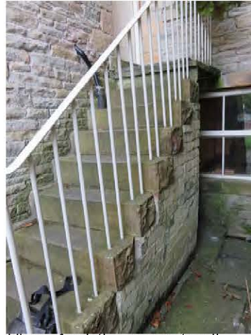
View of existing support wall below rear steps.
