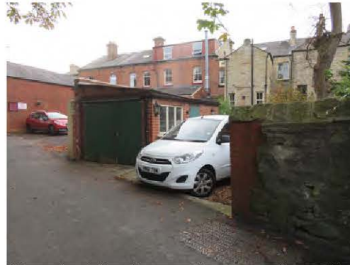
View of existing Garage, from rear alley, with roof heights of adjacent properties shown in context.
