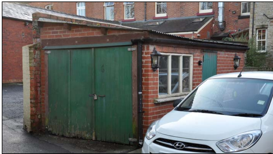
Existing garage, facing onto back street
