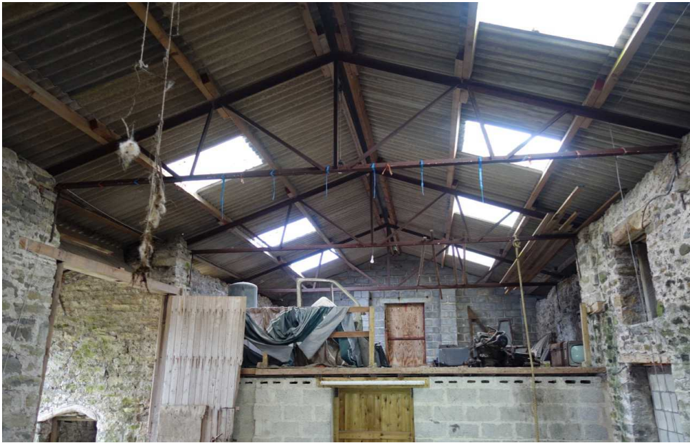
Interior of stone Barn D
