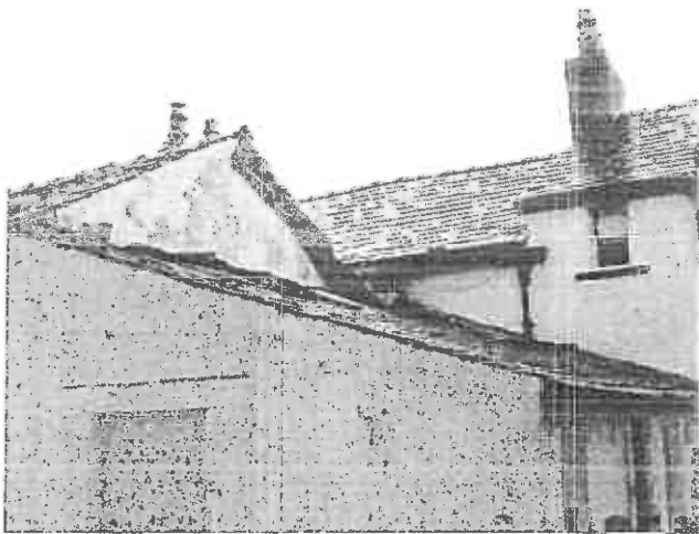
Target Note 4: Rear elevation of pub with moderate - high bat roost potential due to various roof access points.
