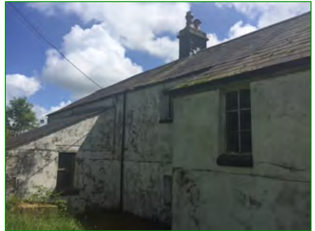
The northwest elevation of the farmhouse
