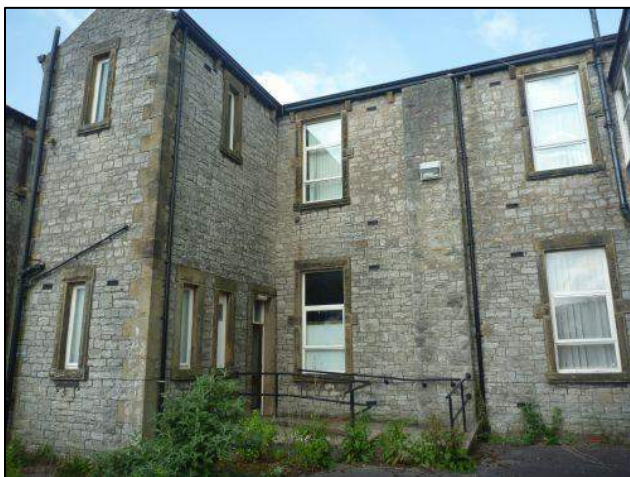
Photo 29: Building 3, southern elevation, middle
