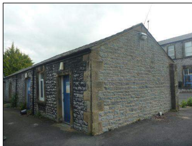
Photo 36: Building 4, western and northern elevation, western end
