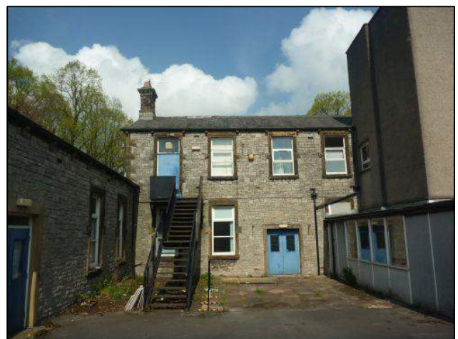
Photo 6: Building 1, southern elevation
