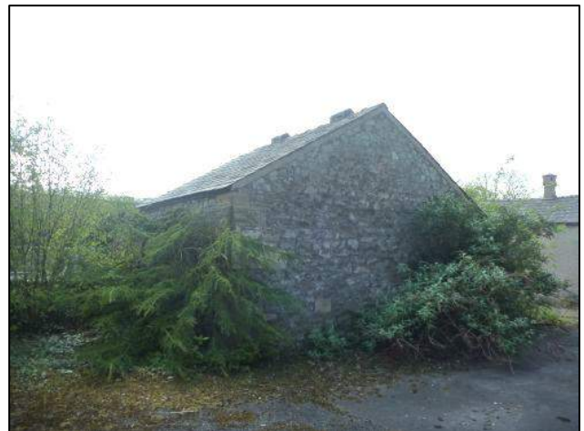
Photo 42: Building 6, northern and eastern elevations
