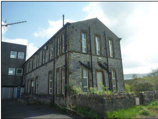
Photo 27: Building 3, northern and western elevations
