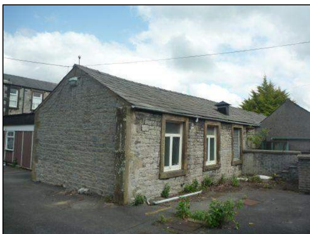
Photo 35: Building 4, western and southern elevations
