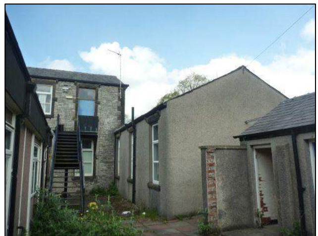
Photo 12: Building 1, southern elevation, eastern end
