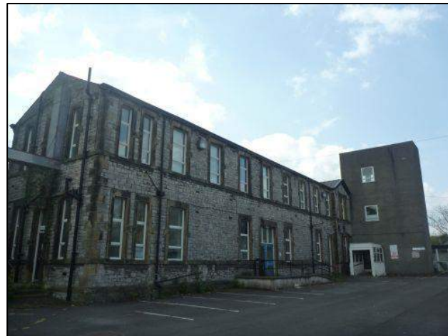
Photo 32: Building 3, northern elevation, eastern end
