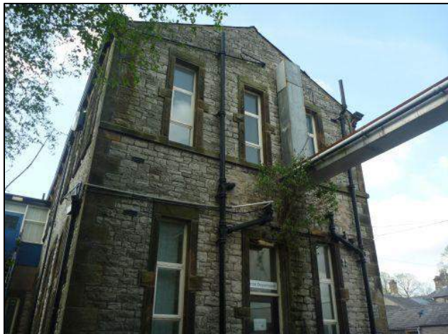
Photo 31: Building 3, eastern elevation
