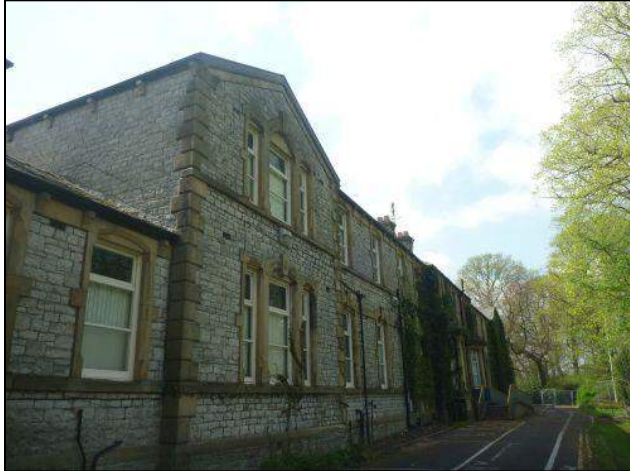
Photo 1: Building 1, northern elevation, eastern end
