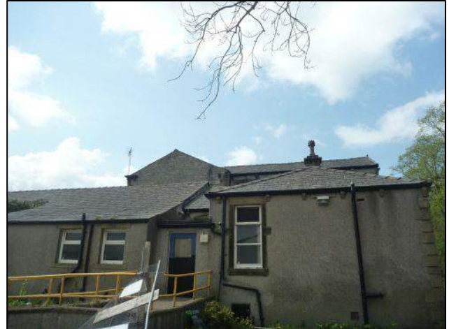
Photo 14: Building 1, eastern elevation, northern end
