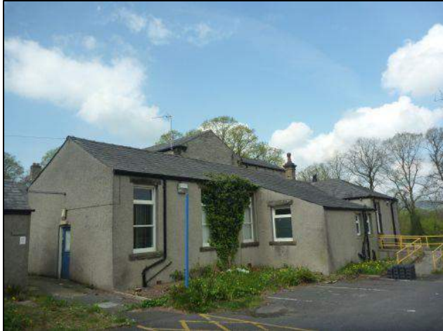
Photo 13: Building 1, eastern elevation, southern end
