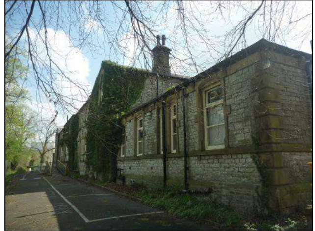
Photo 2: Building 1, northern elevation, western end
