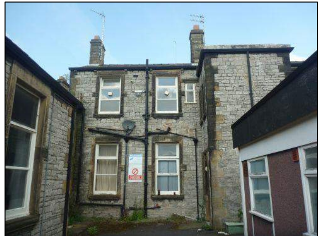
Photo 10: Building 1, southern elevation
