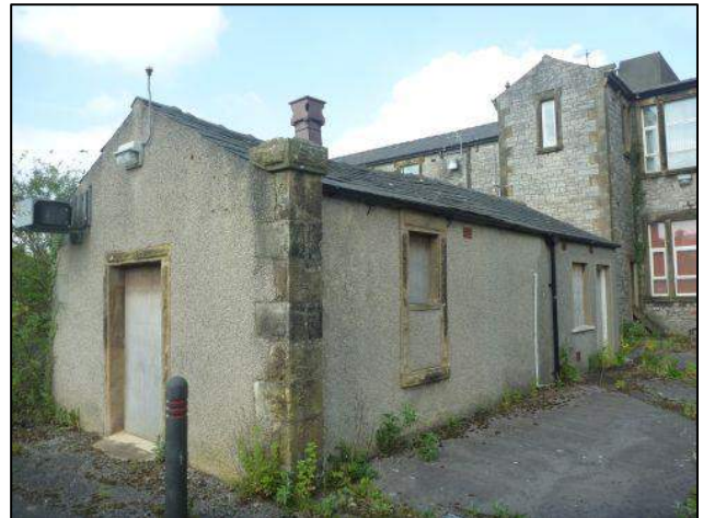
Photo 40: Building 5, southern and eastern elevations
