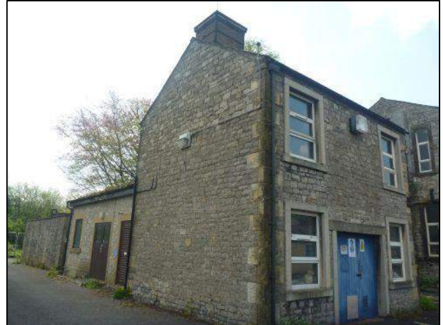
Photo 44: Building 7, eastern elevation
