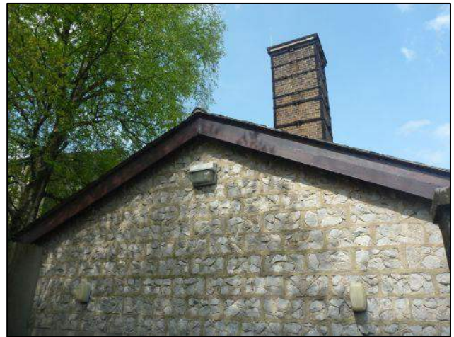
Photo 46: Building 7, southern elevation
