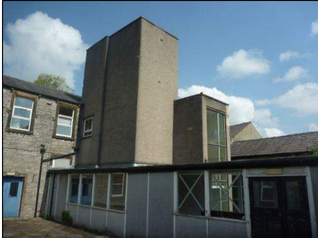
Photo 7: Building 1, southern elevation (including section of covered walkway in the foreground)
