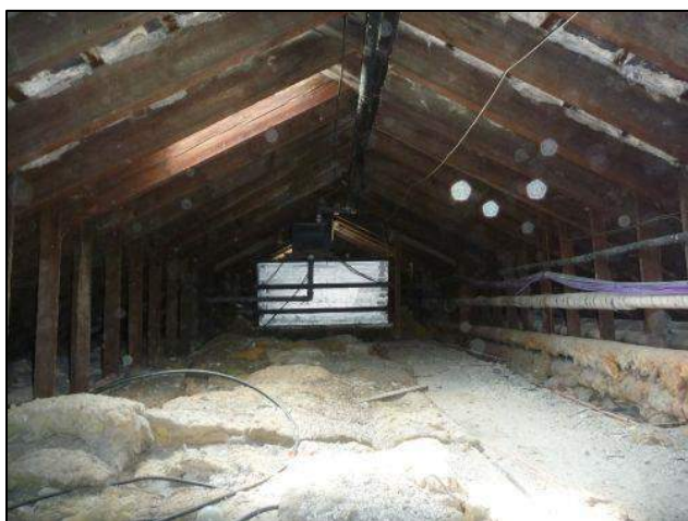
Photo 33: Building 3, roof void.
