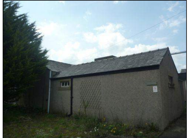
Photo 38: Building 4, northern and eastern elevations
