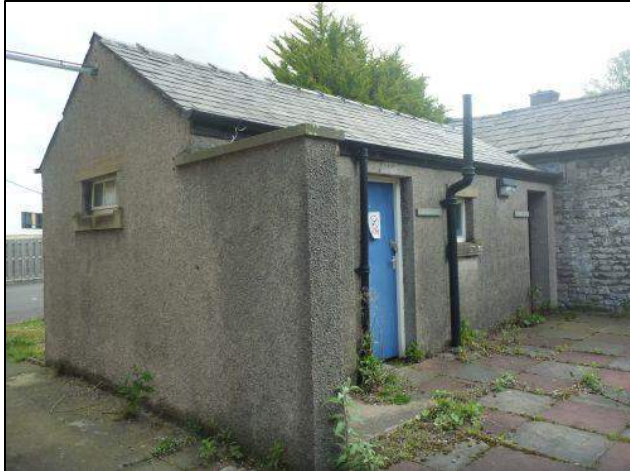
Photo 37: Building 4, northern and western elevations, eastern end
