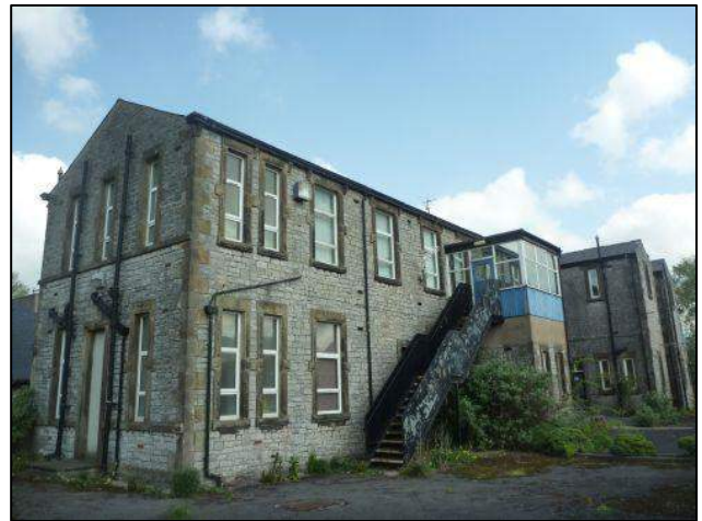
Photo 28: Building 3, southern elevation, western end
