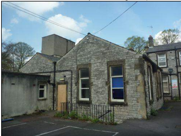
Photo 9: Building 1, southern elevation
