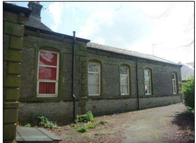
Photo 4: Building 1, western elevation, southern end
