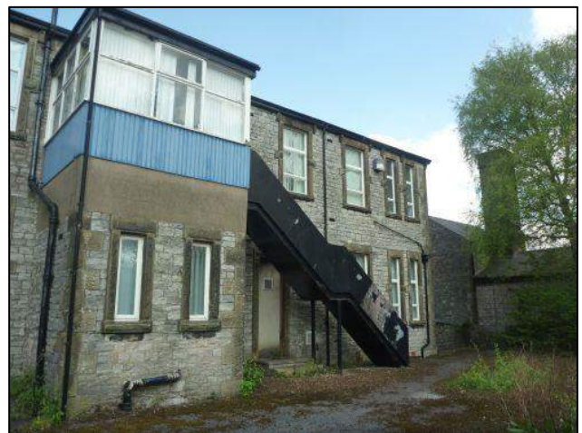
Photo 30: Building 3, southern elevation, eastern end
