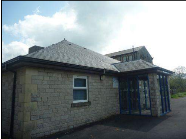
Photo 25: Building 2, western elevation
