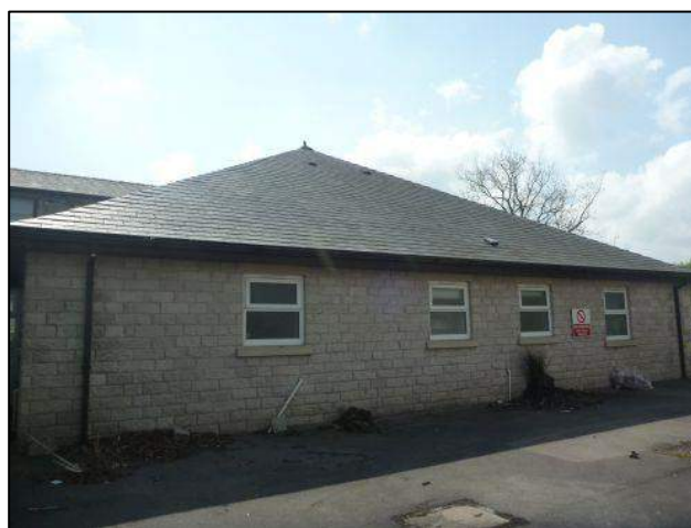
Photo 24: Building 2, northern elevation
