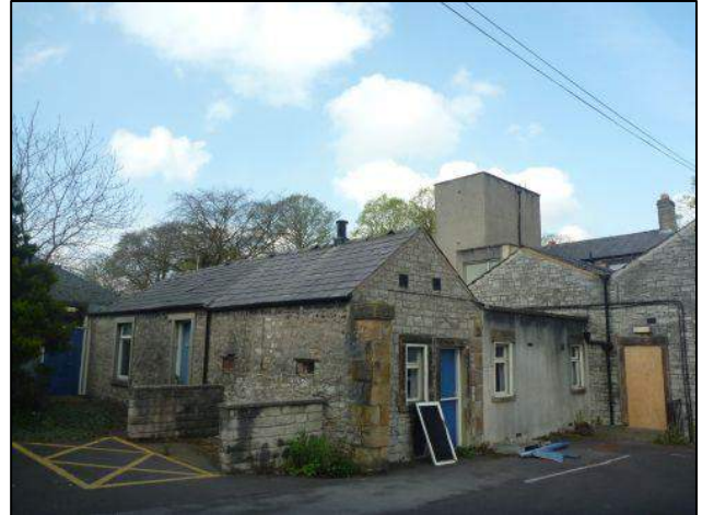
Photo 8: Building 1, southern elevation
