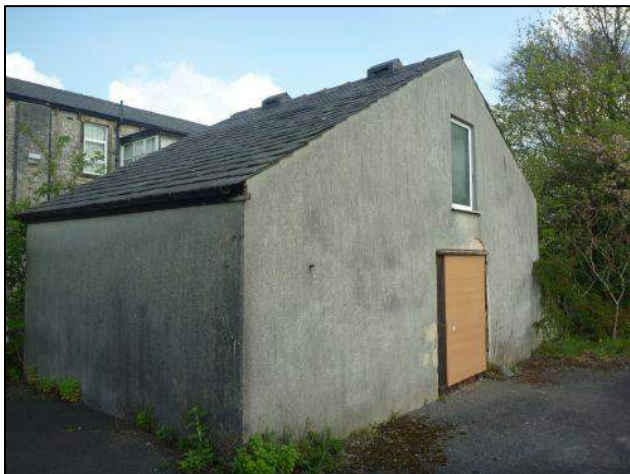
Photo 41: Building 6, southern and western elevations
