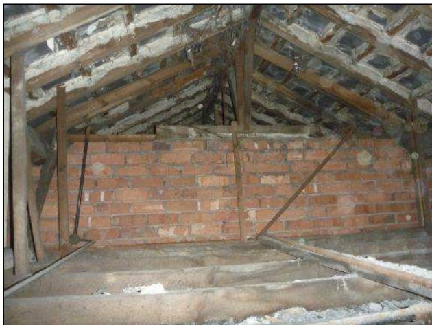
Photo 17: Building 1, roof void above single-storey section at south-western corner (1b)
