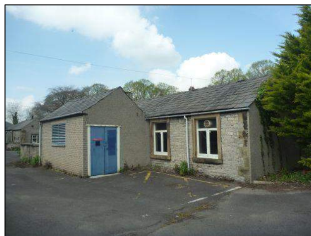
Photo 34: Building 4, southern elevation
