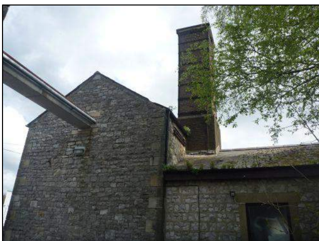
Photo 47: Building 7, western elevation
