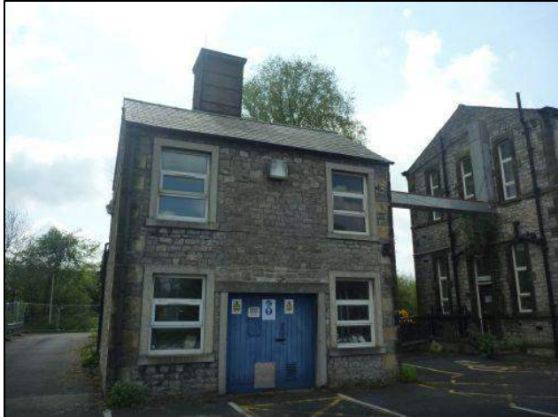
Photo 43: Building 7, northern elevation
