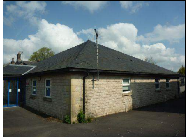
Photo 26: Building 2, southern elevation
