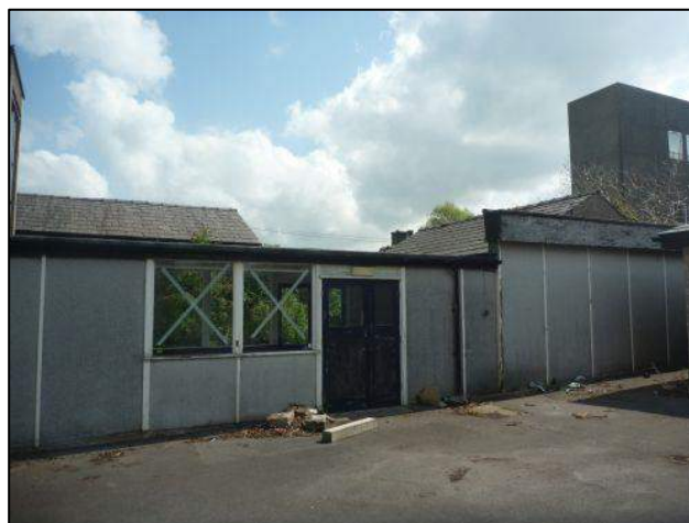
Photo 22: Western elevation of covered walkway which joins Buildings 1, 2 and 3
