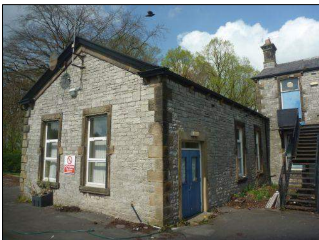
Photo 5: Building 1, southern elevation, western end
