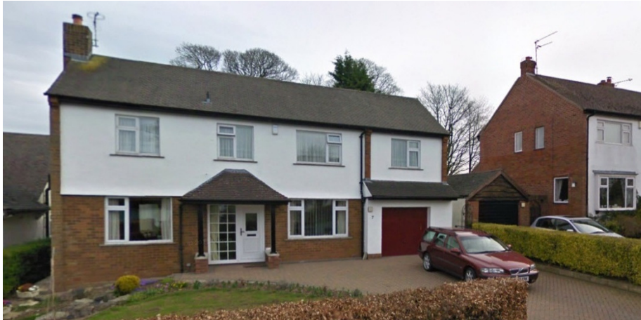
View of detached property close to the site
