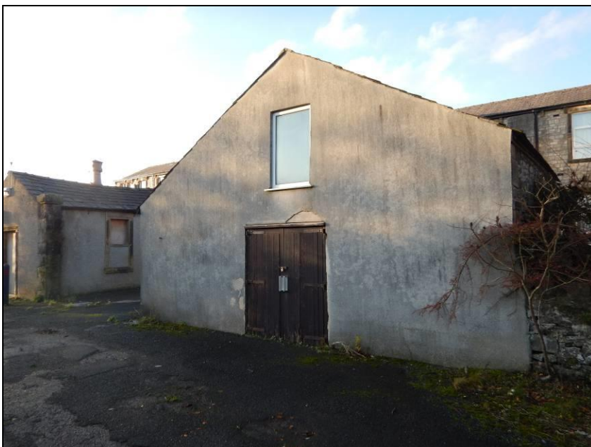
Photograph 13: Gardner's store (R) and mortuary (L) at rear of former Infirmary.
