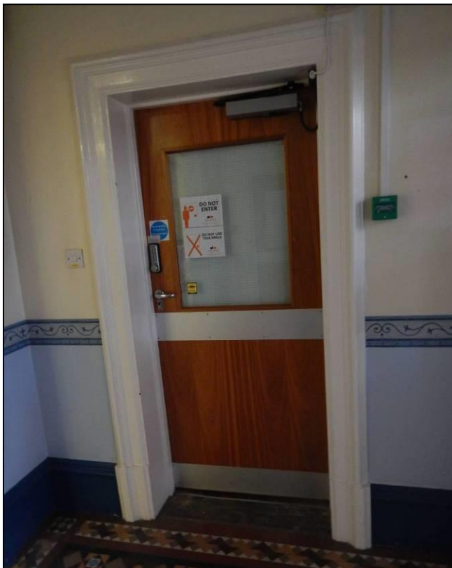
Photograph 6: Original door architrave.
