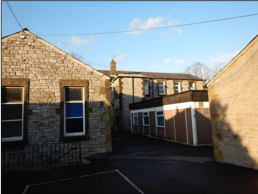
Photograph 2: Rear elevation of former Workhouse with single-storey outshot (kitchens) on the left and smaller two-storey outshot and modern prefabricated building to the right.
