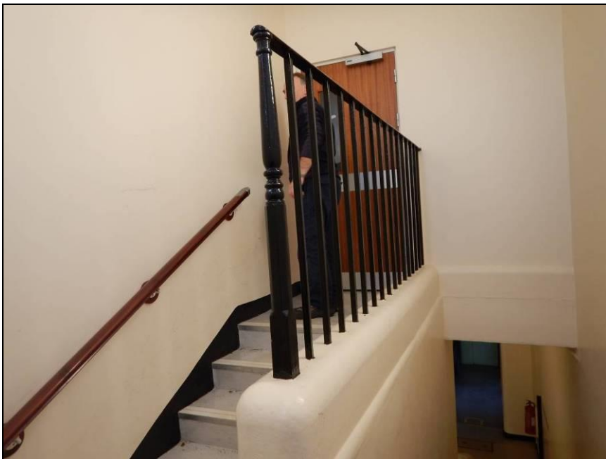
Photograph 10: Historic stair balustrade
