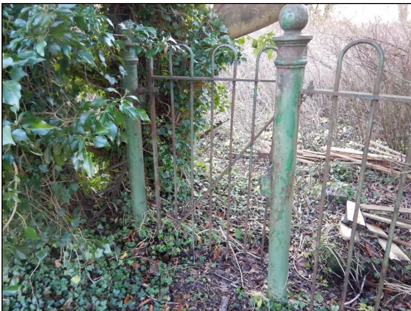
Photograph 18: Railings and gate to enclosed front area at west of site.
