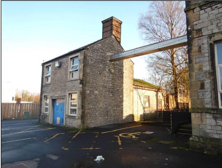
Photograph 14: Boiler house with later brick chimney.
