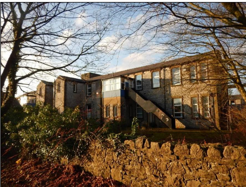
Photograph 9: Rear elevation of the former Infirmary with gabled outshots to the left and the right rectangular outshot with modern fire escape to the right of the photograph.
