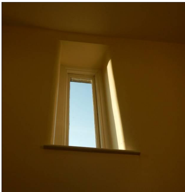
Photograph 11: Curved openings to window.
