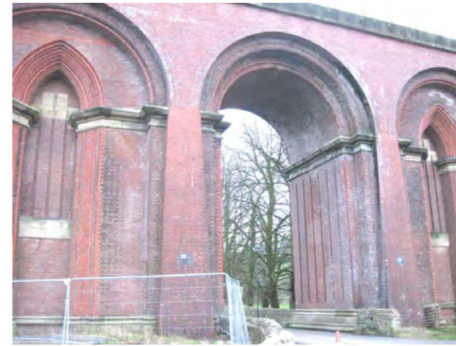
View from Cross House towards viaduct feature arches
