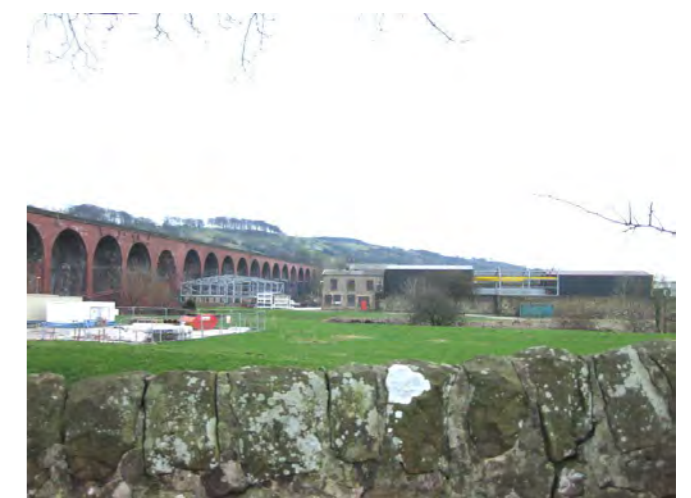
View from East Ridding Lane towards the river and The Nab
