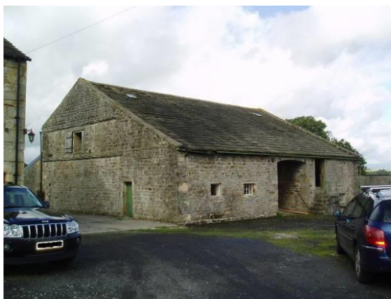
South elevation with wagon entrance
