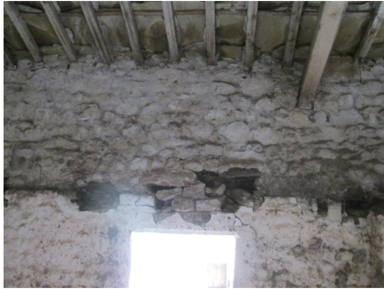
Photo 14 – Holes in Front Wall where First Floor Removed
