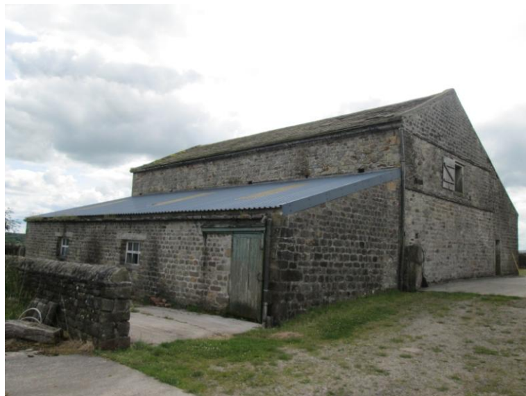
Photo 2 – Rear of Barn
