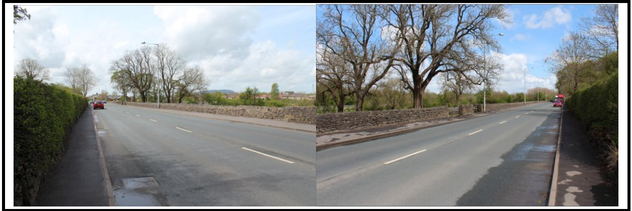
View to exiting access point
