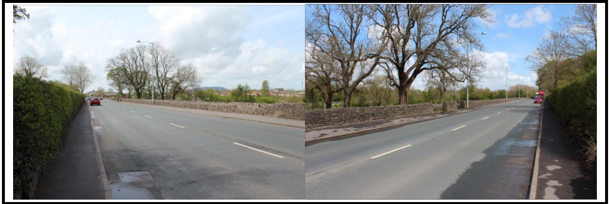
View to exiting access point
