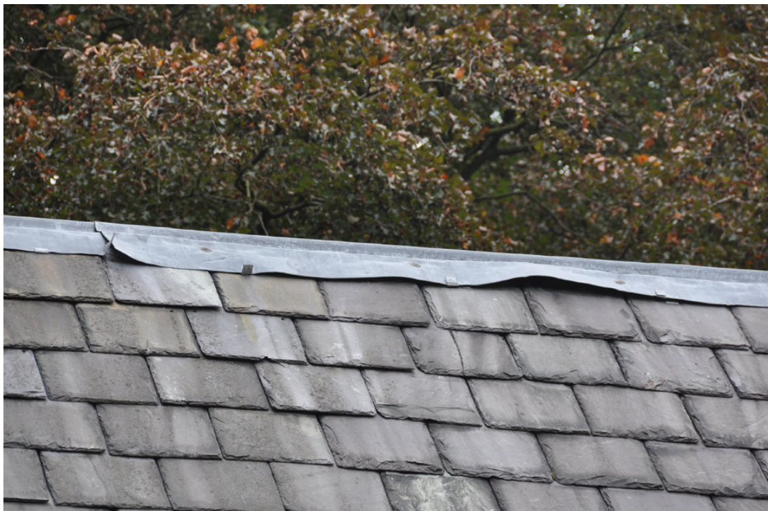
Garnet House – raised lead on ridge (potential bat roost feature). September 2014
