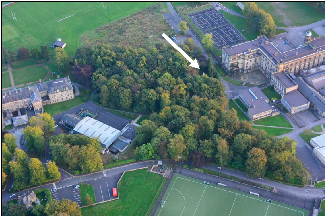
Closer view of proposed development site context – Garnet House marked with white arrow. September 2014.
