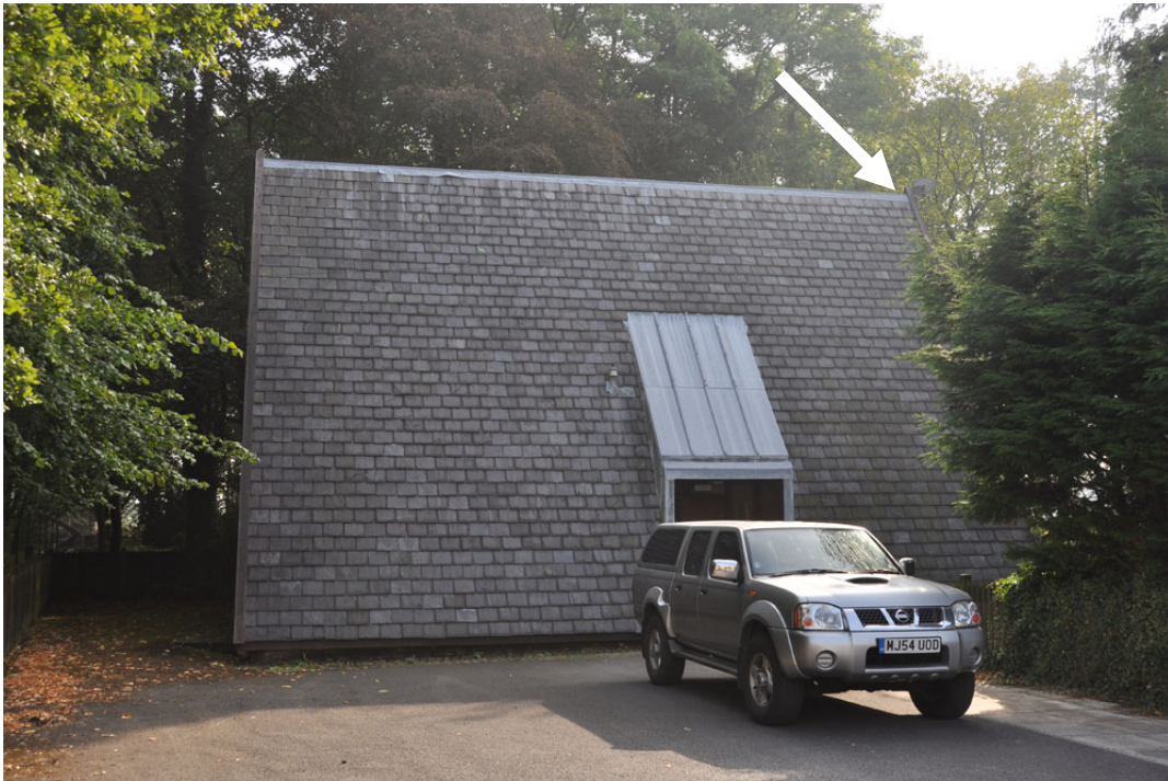
Garnet House (bat roost) – west elevation roof pitch. Arrow denotes bat emergence point in 2017. May 2017
