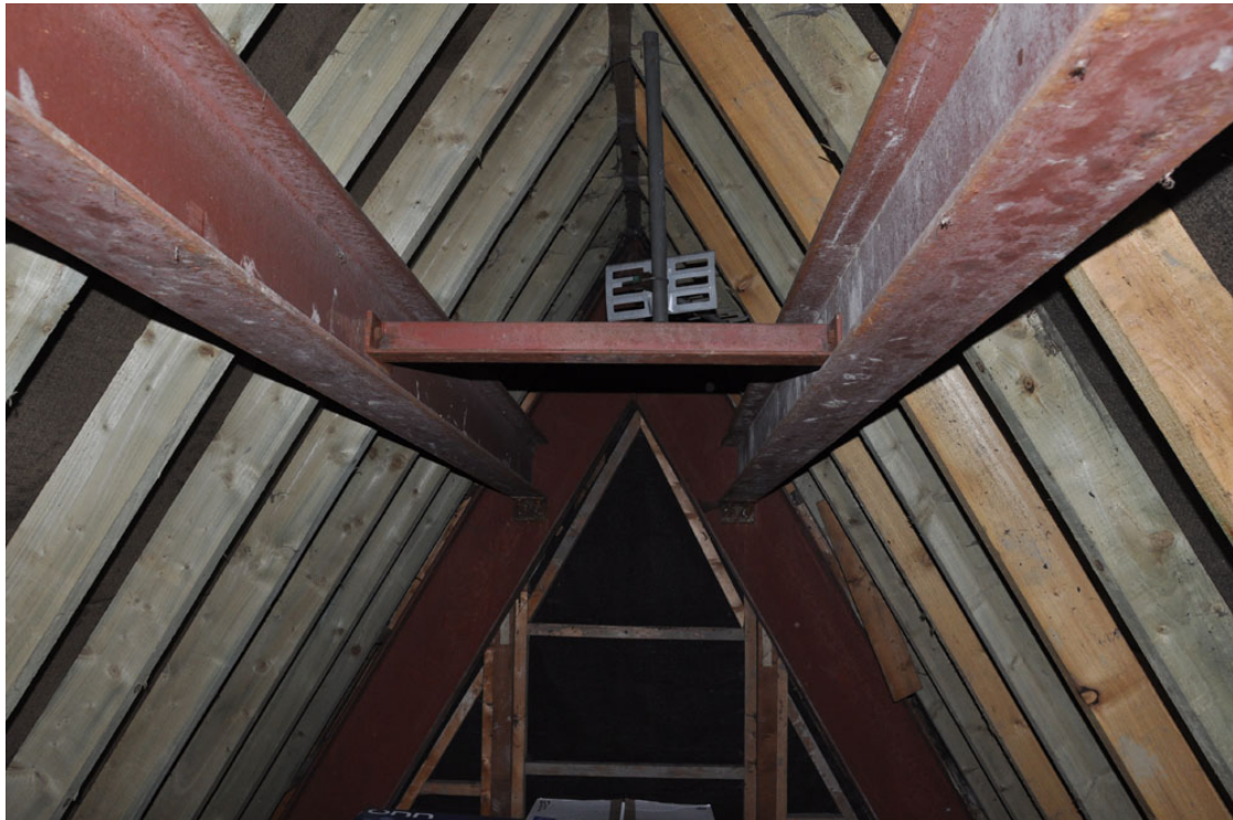
Internal view of Garnet House roof void. September 2014
