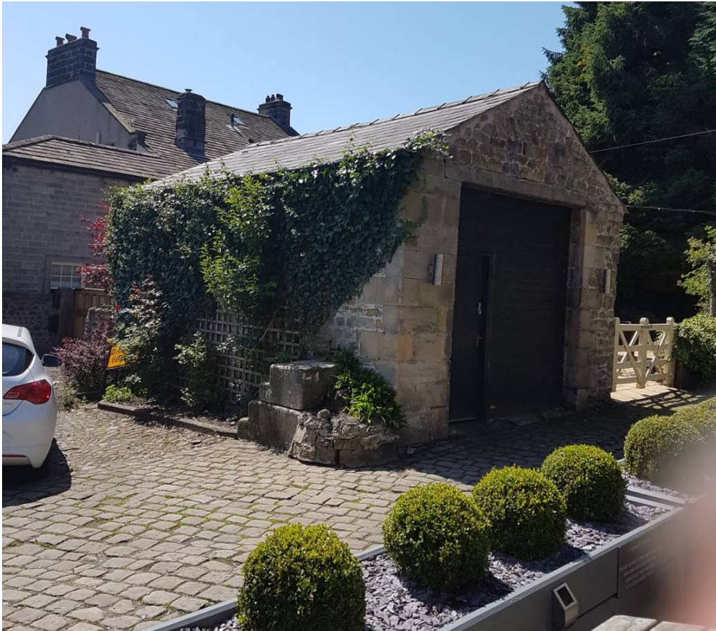
west elevation of detached store building
