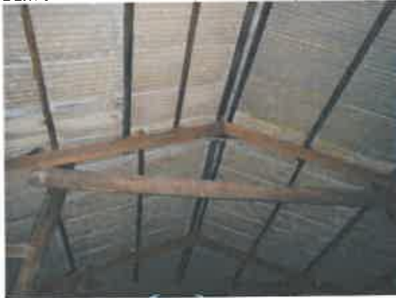
Barn 3 Timber stanchions, trusses and purlins
