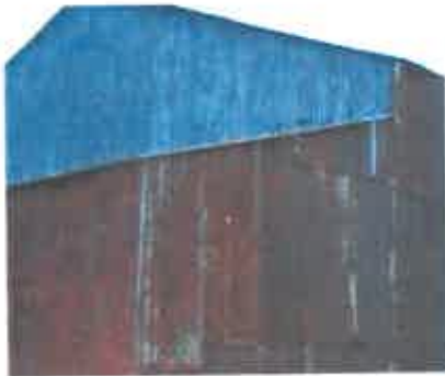
Barn 3 corrugated steel sheet fixed over timber frame.
