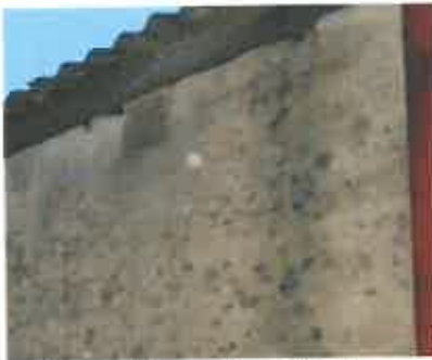
Barn 1 with corrugated fibre cement sheet walls and cast concrete base walls, concrete portal frame.
