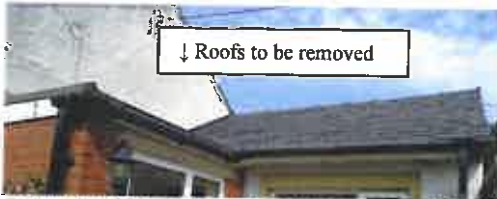
The side porch with pitched slate roof and felt flat
