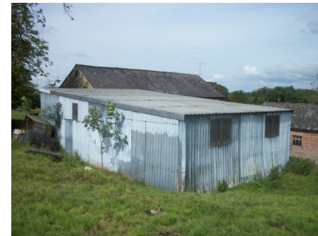
Figure 7: Building B - rear elevation
