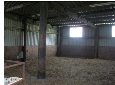
Figure 10: view inside Barn B
