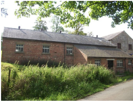
Figure 3: Brick shippon – building C
