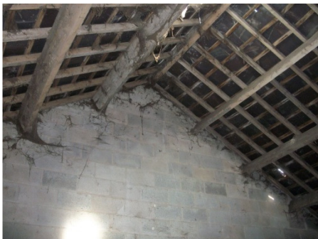
Figure 9: Barn A - roof detail
