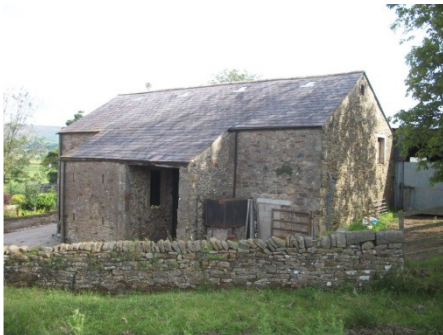
Figure 6: Stone barn - building A
