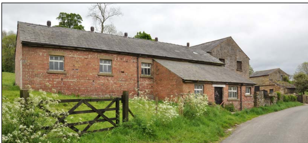
Photo 1: Farm buildings group, from the north
