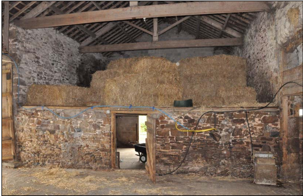
Photo 6: Barn interior with wall enclosing shippon
