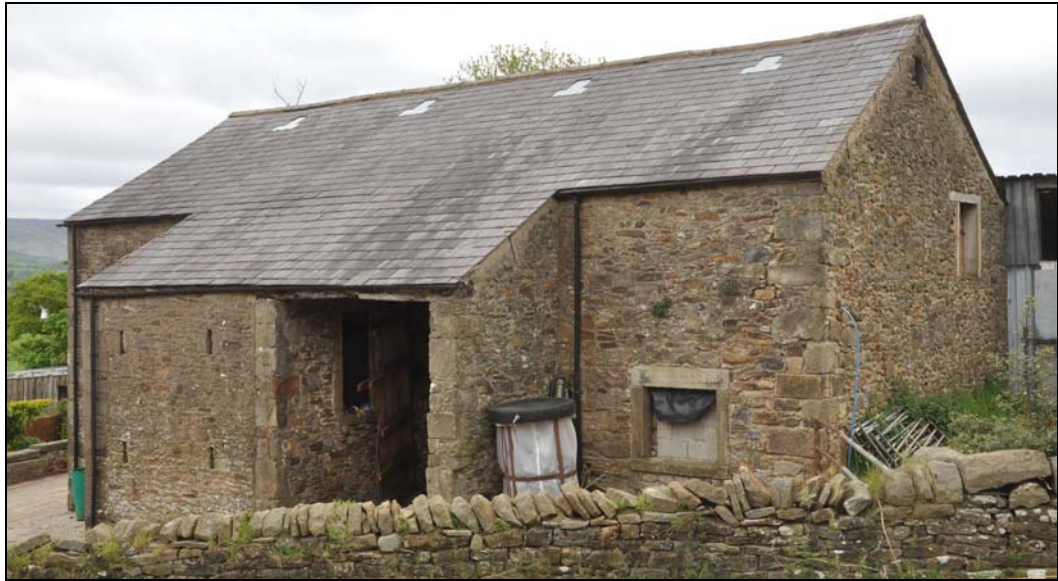
Photo 3: Front of barn
