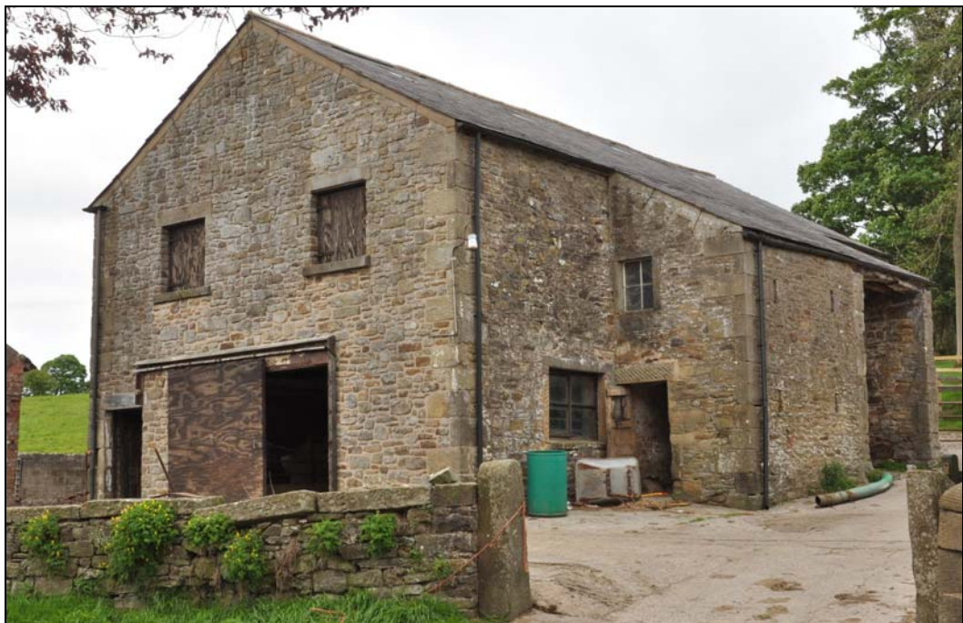
Photo 2: Front of barn and rebuilt gable
