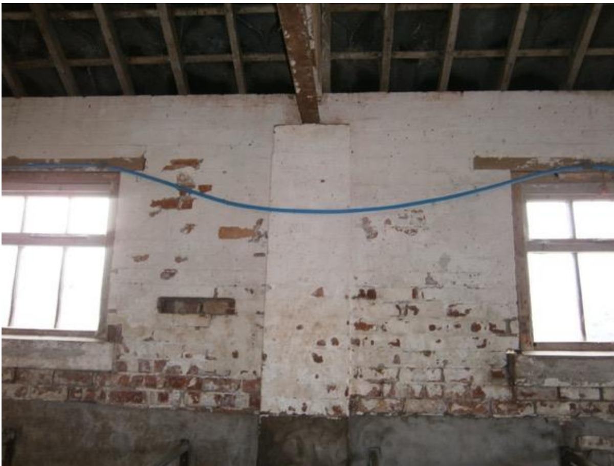
Photo 22 - Internal main section – showing buttress to beams
