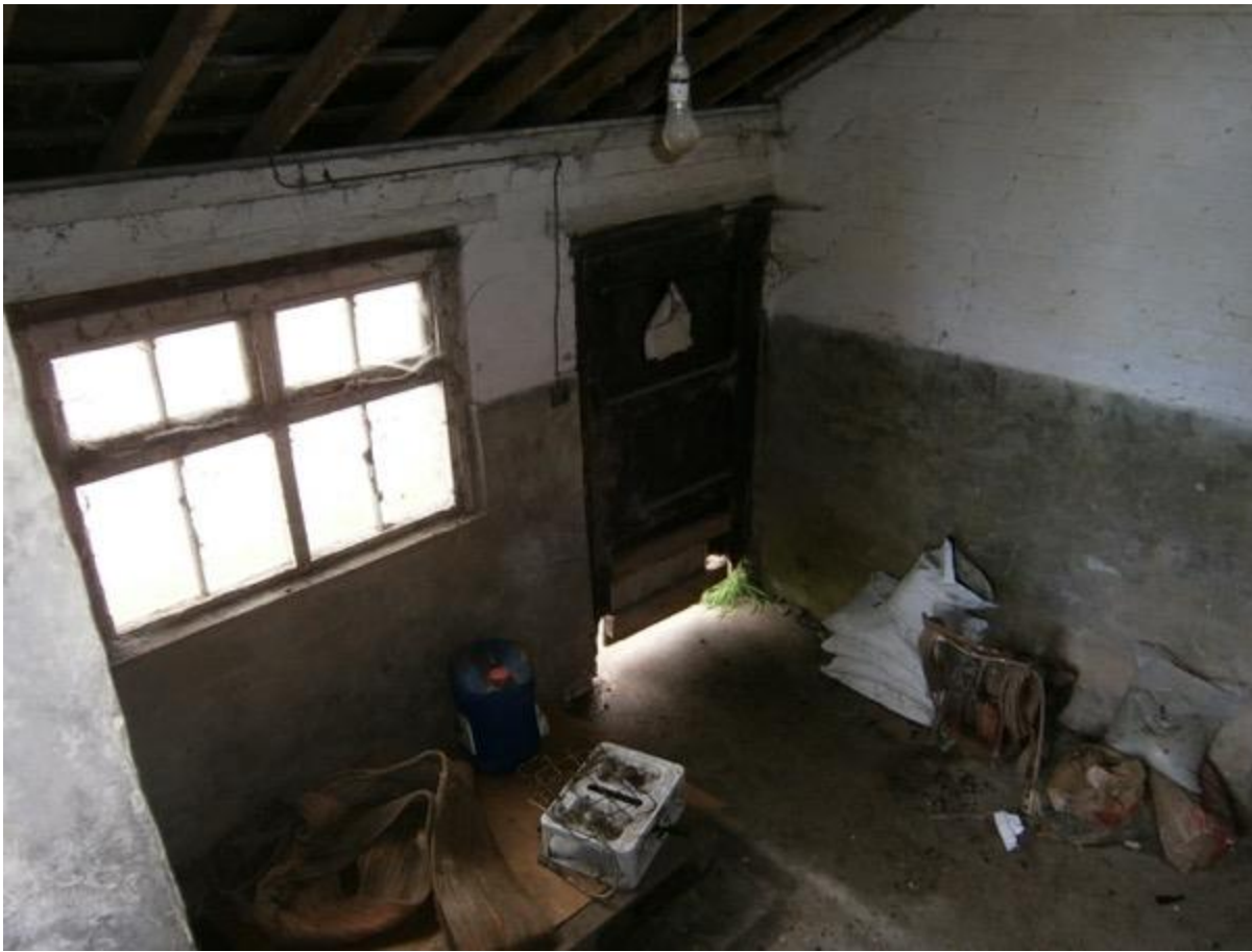
Photo 17 - Internal of lean-to section
