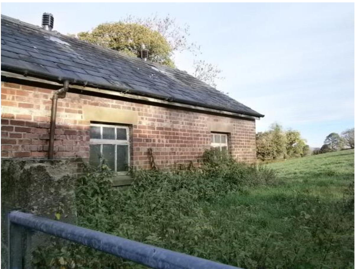
Photo 8 – South East Elevation
