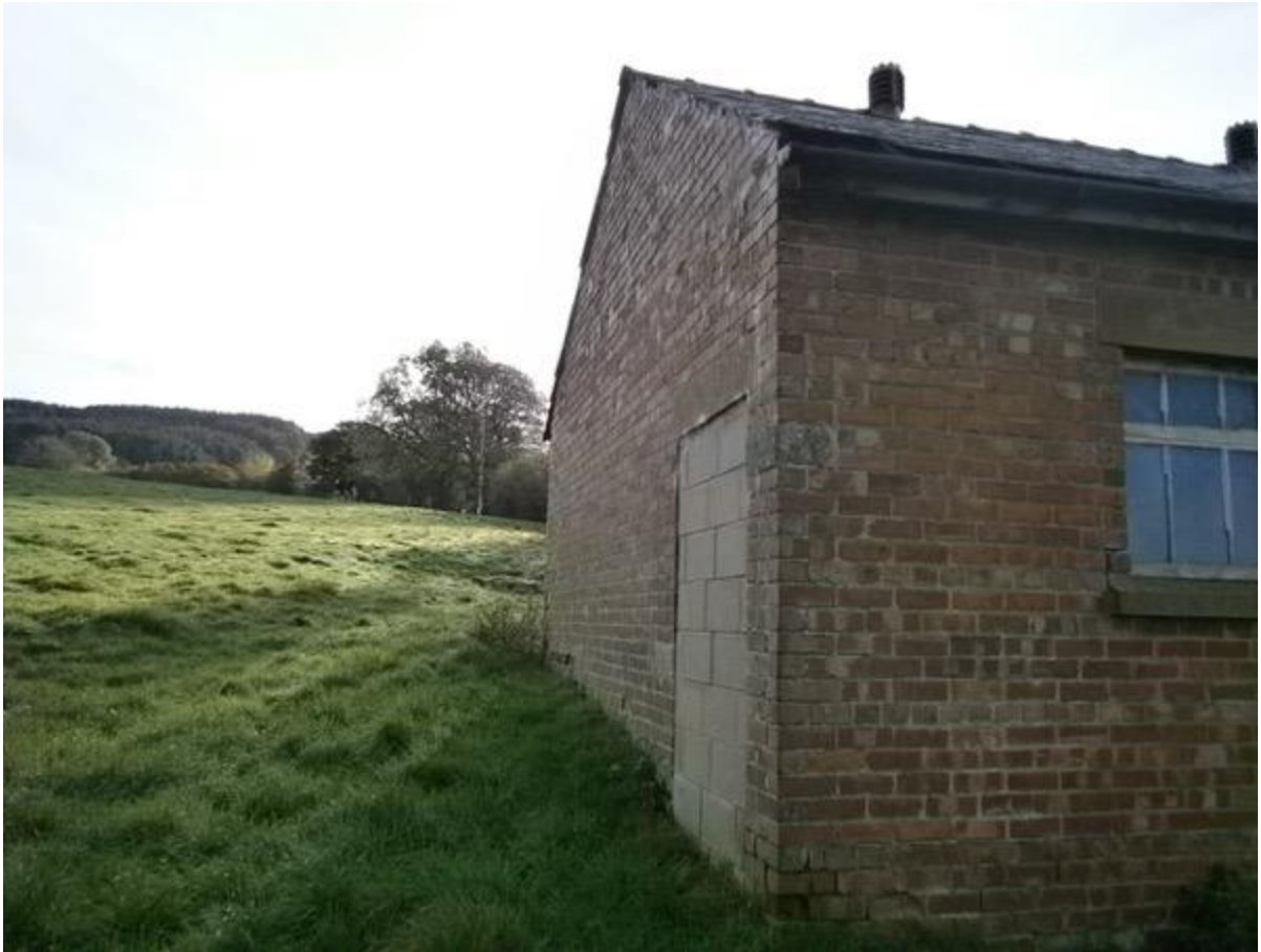
Photo 14 - North East Elevation
