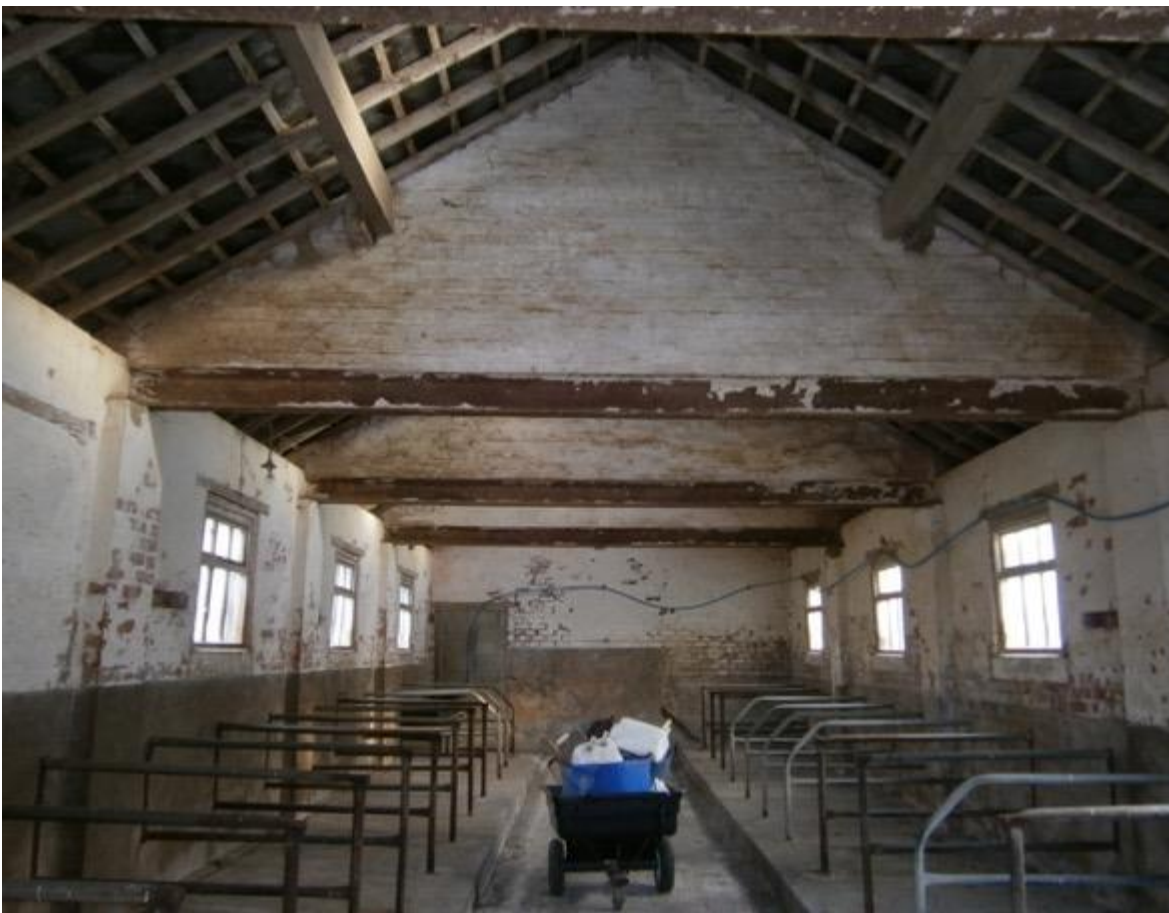
Photo 20 – Internal main section
