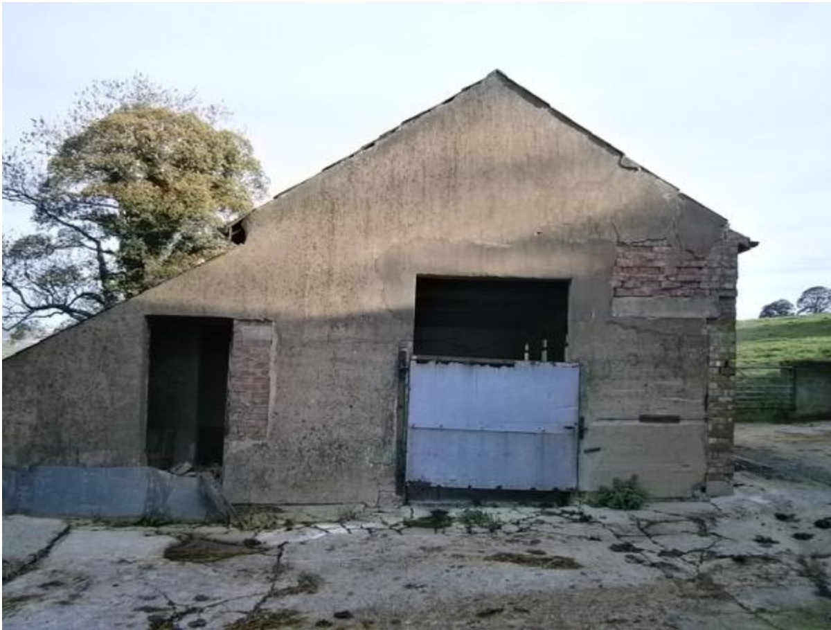
Photo 1 - South West Elevation
