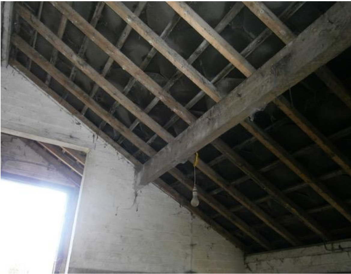
Photo 19 – Roof to lean-to section
