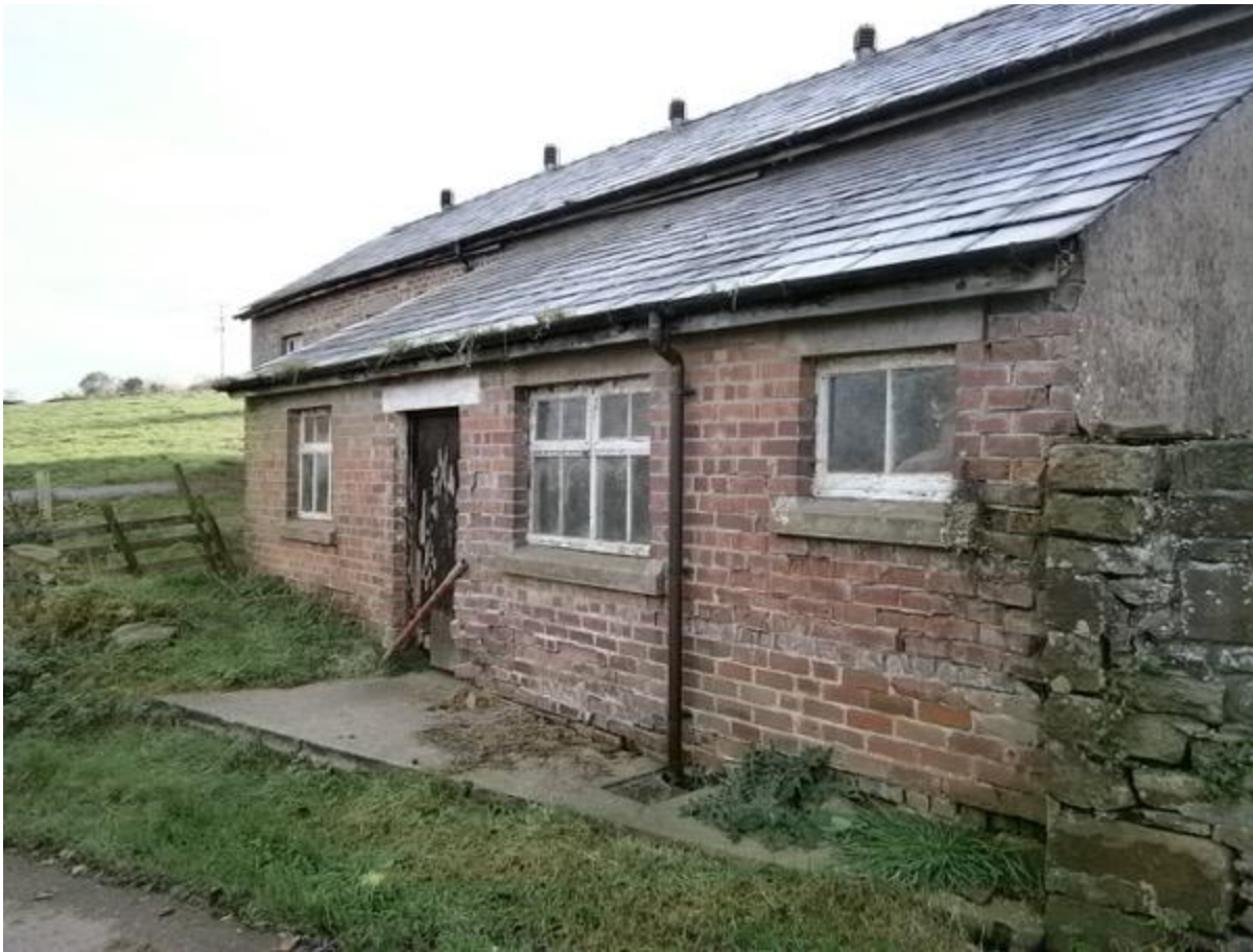
Photo 10 – North West Elevation
