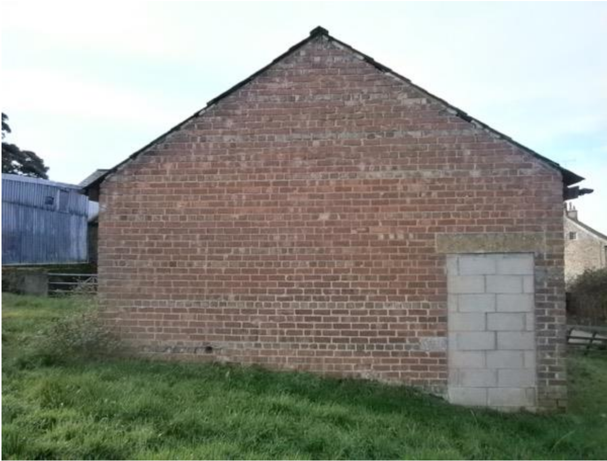
Photo 15 - North East Elevation
