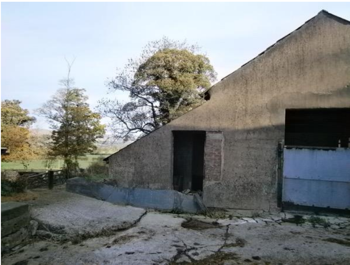
Photo 2 – South West Elevation
