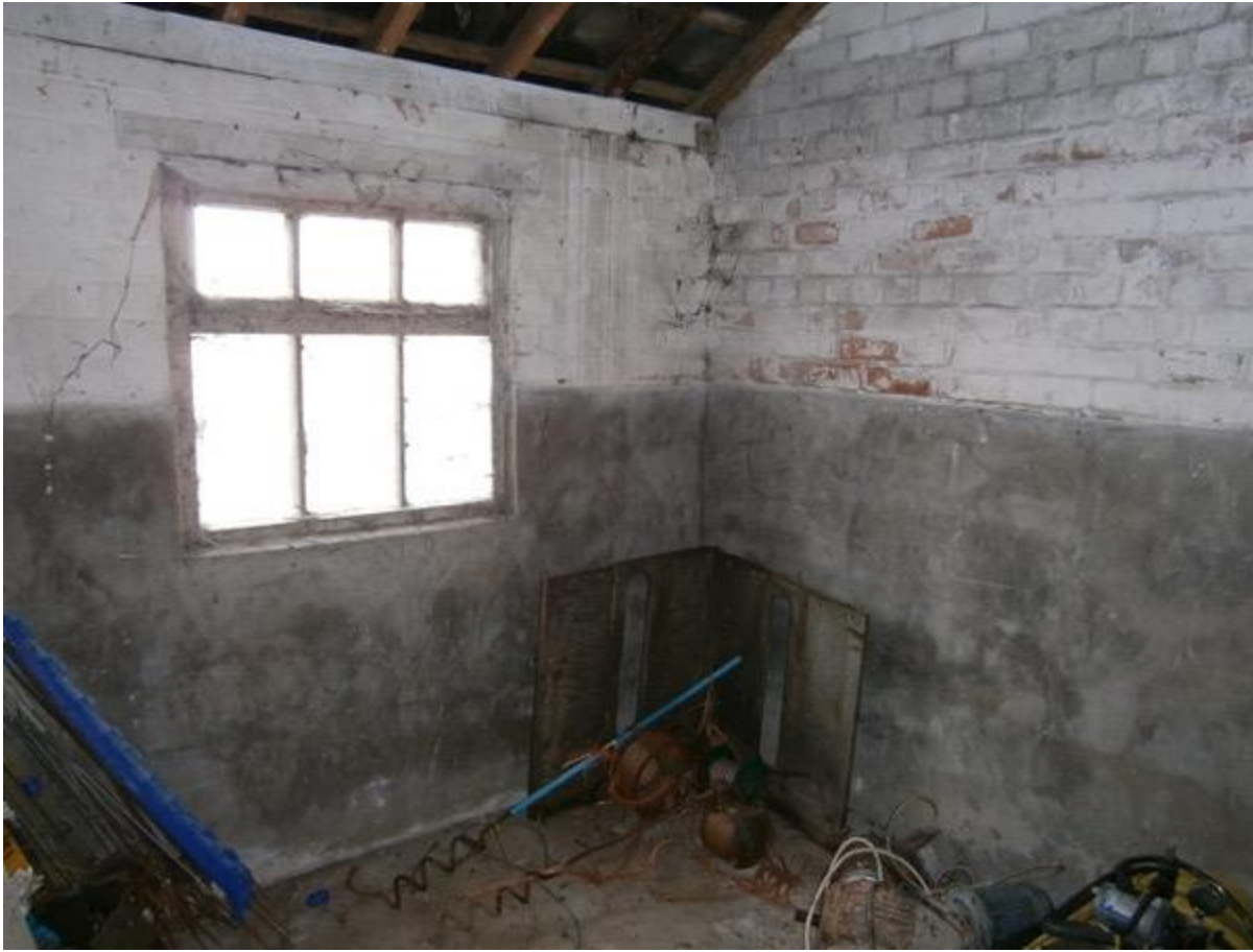
Photo 18 - Internal of lean-to section
