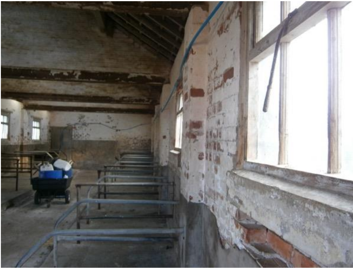
Photo 21 - Internal main section
