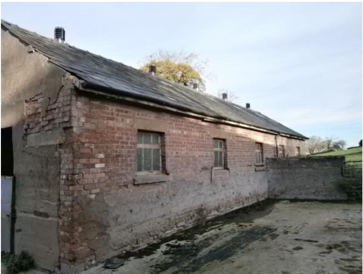
Photo 6 – South East Elevation
