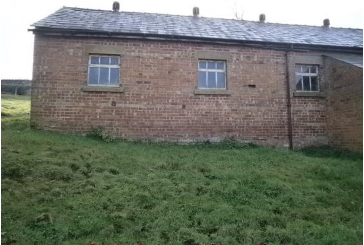
Photo 13 - North West Elevation
