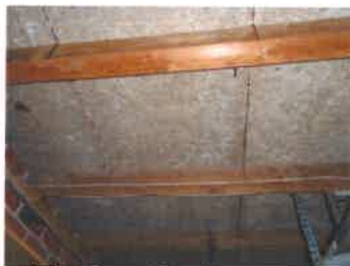
underside of garage flat roof
