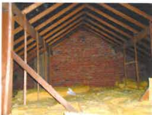
House roof void
