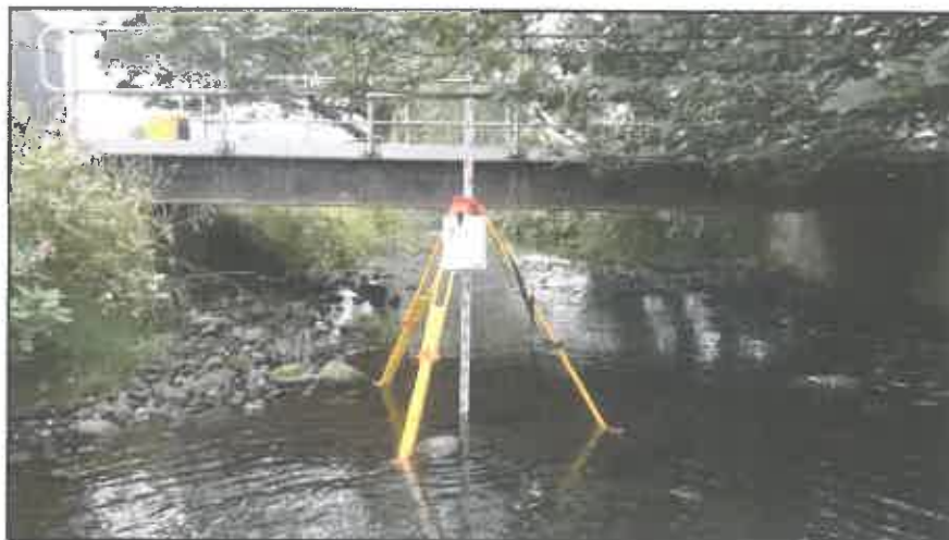
Figure 3-5: Bridge to Chipping WWTW
