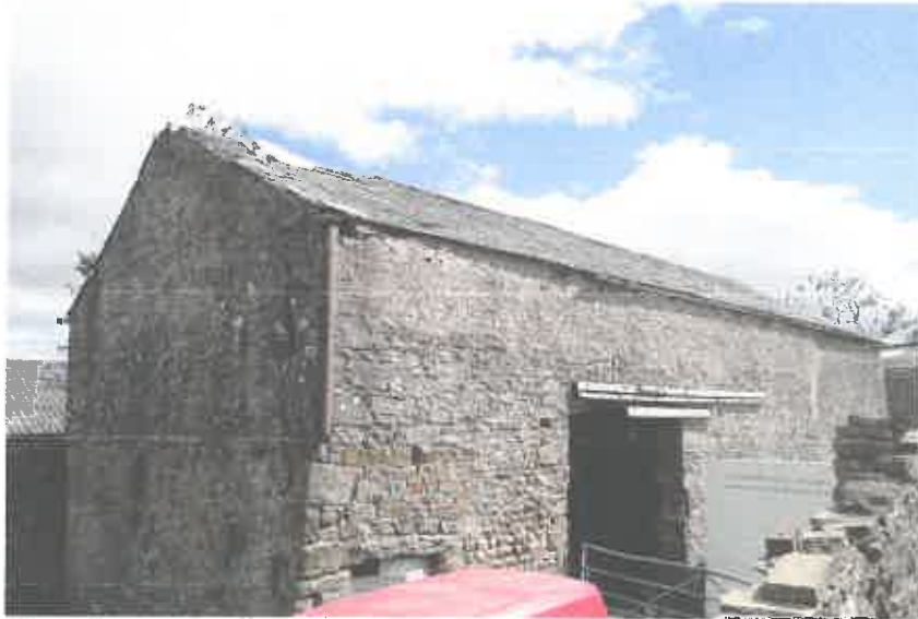
3 - A traditional stone built and slate roofed barn. Gaps and crevices are present in the external and internal walls. Roof slates are unlined and lifted tiles and missing tiles present. The building can be considered of high potential for roosting bats.
