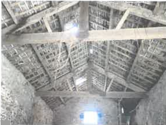
3 - A traditional stone built and slate roofed barn. Gaps and crevices are present in the external and internal walls. Roof slates are unlined and lifted tiles and missing tiles present. The building can be considered of high potential for roosting bats.
