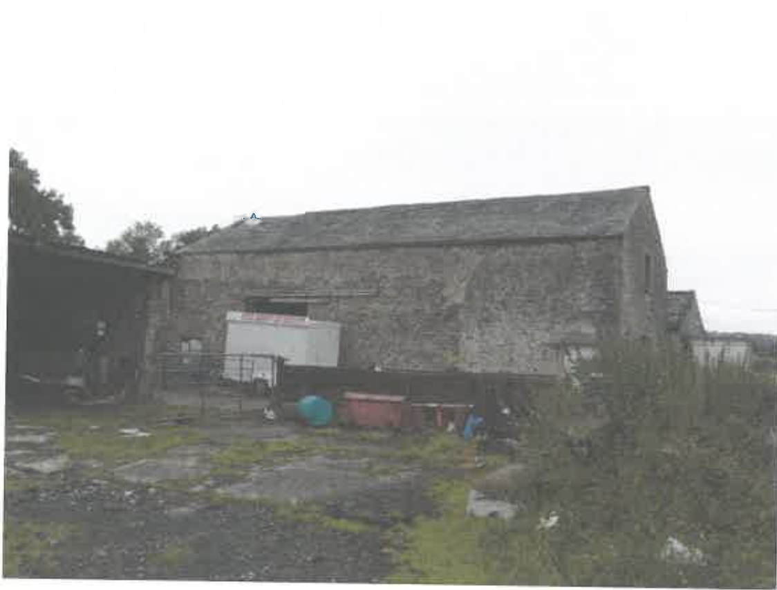
1 : Photo of the front elevation.
