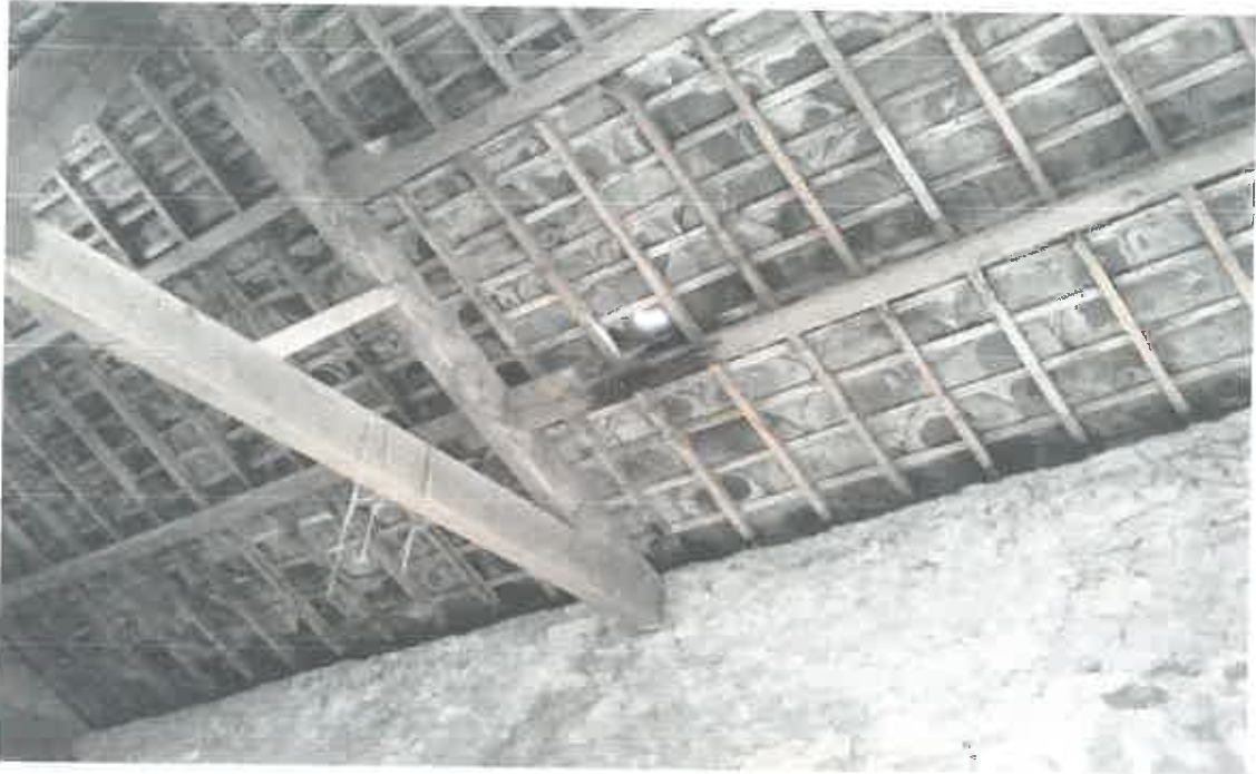
5b : Photo of internal roof structure – West gable end
