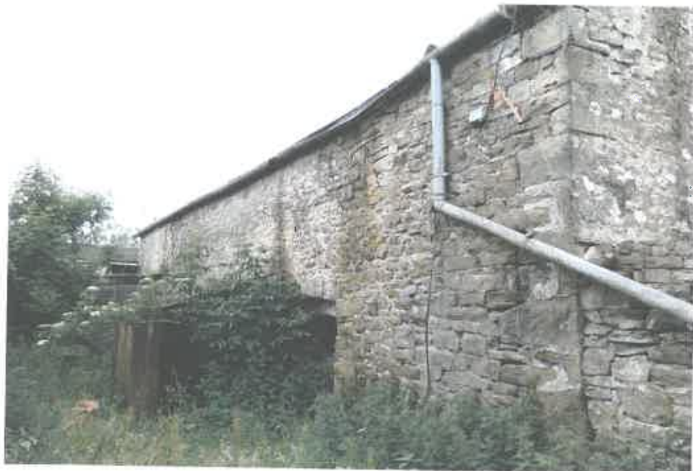
2b : Photo of Step in rear elevation masonry
