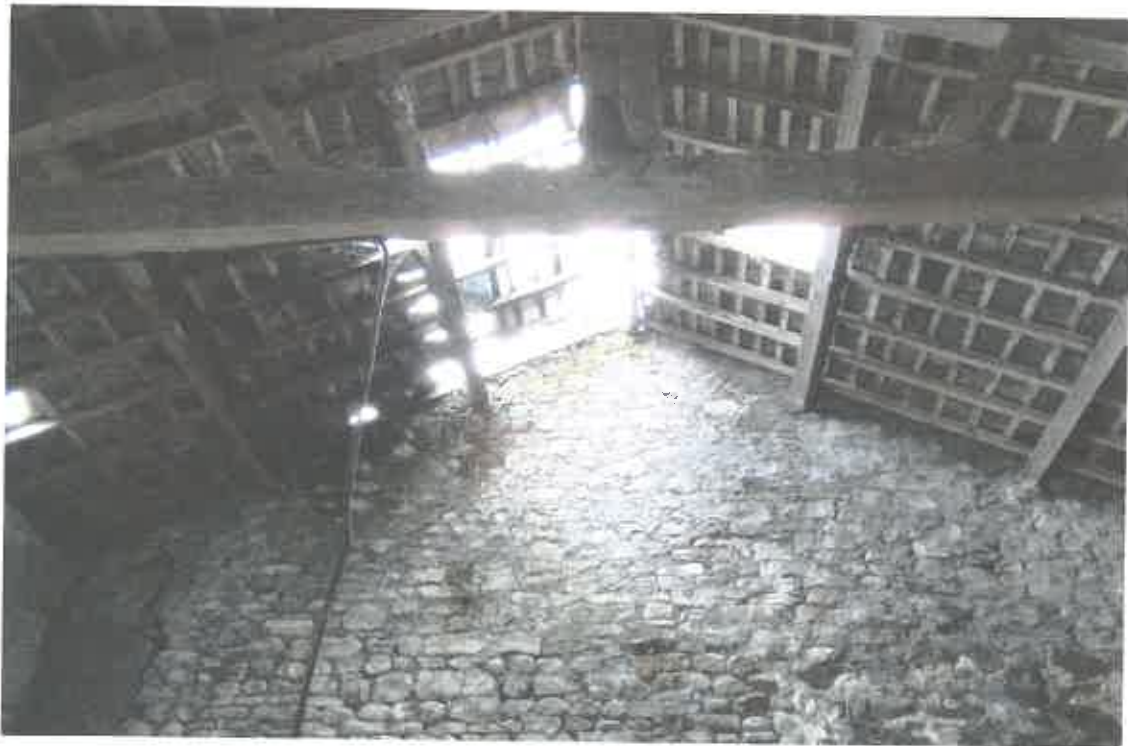
5a : Photo of internal roof structure – East gable end
