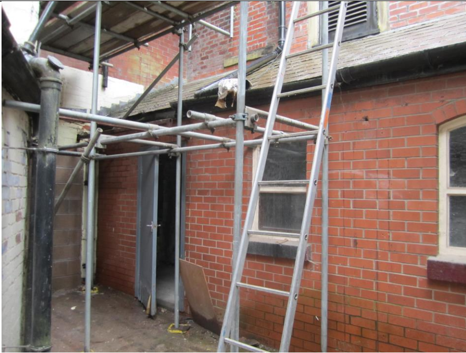
4 Existing modern lean-to within the rear courtyard.
