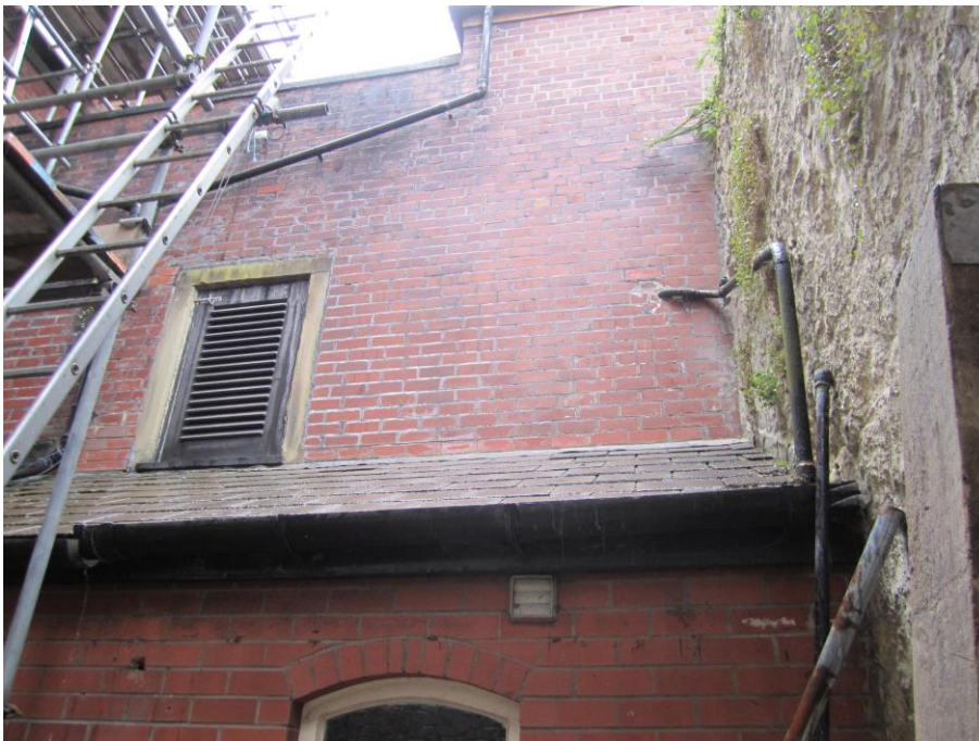
5 Two storey high stone retaining wall enclosing the rear yard.
