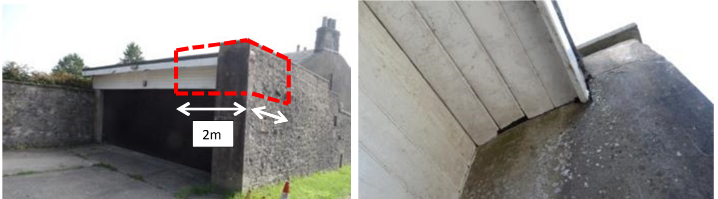
Figure 16: Critical area of garage roof requiring hand removal of materials within 2m of the roost area.
