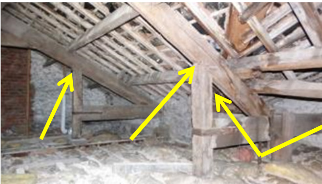
Figure 10: mortice joints provide roost features as shown
