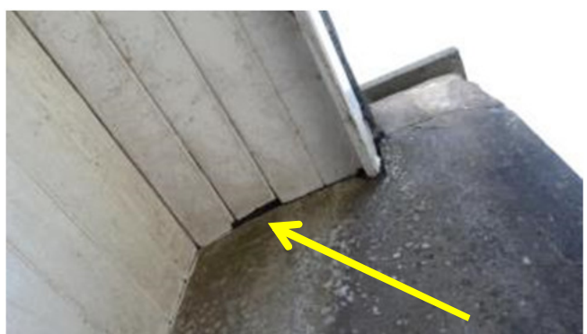
Figure 13: access gap on external wall of garage
