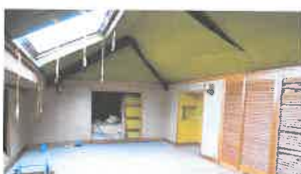
Figure 4: main roof void
