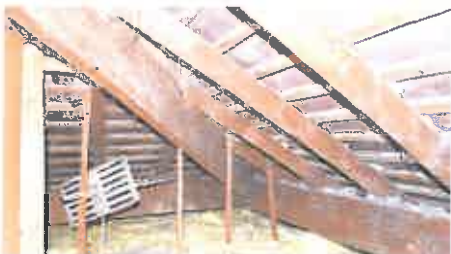
Figure 3: eaves roof void
