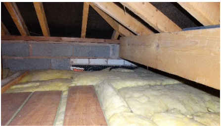
Figure 5: small roof void on side roof pitch
