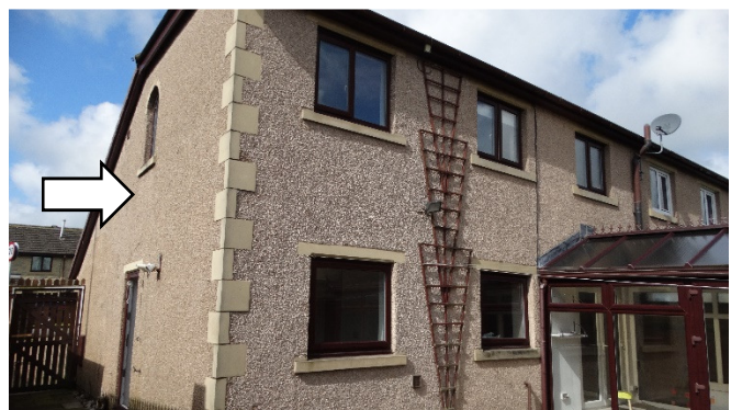
Figure 2: rear and side elevations
