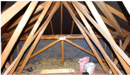
Figure 3: main roof void
