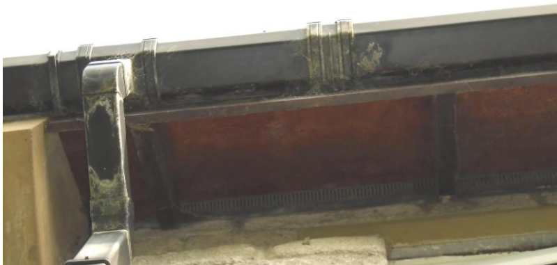
Soffit where the bay window will be positioned
