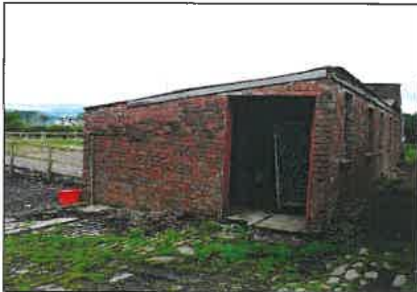
Photo 1: West and south elevation (B1).
