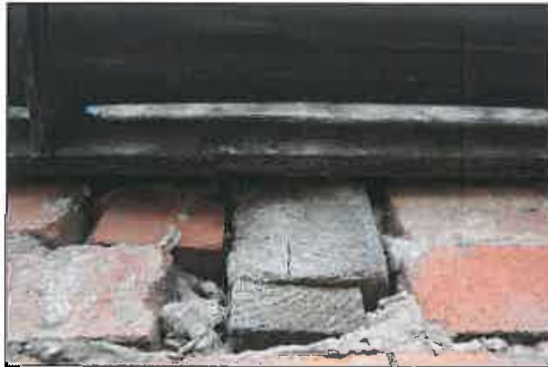
Photo 4: Example of web covered mortar gaps inspected by endoscope.
