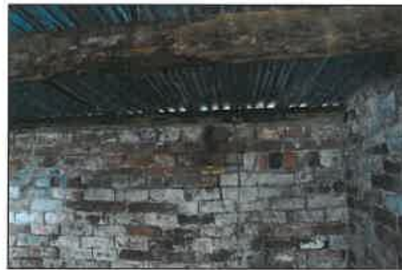
Photo 7: Timber beam at wall tops.
