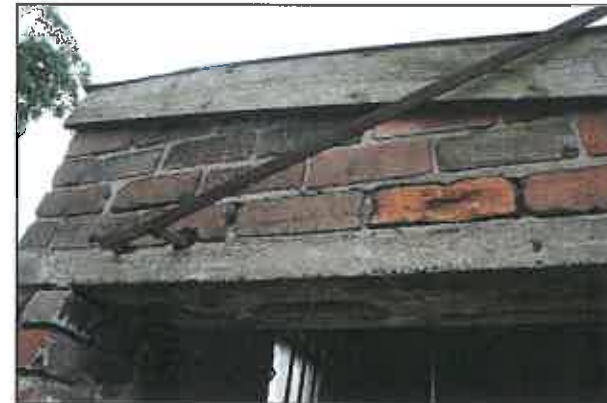
Photo 5: Example of gap to fascia board inspected by endoscope.
