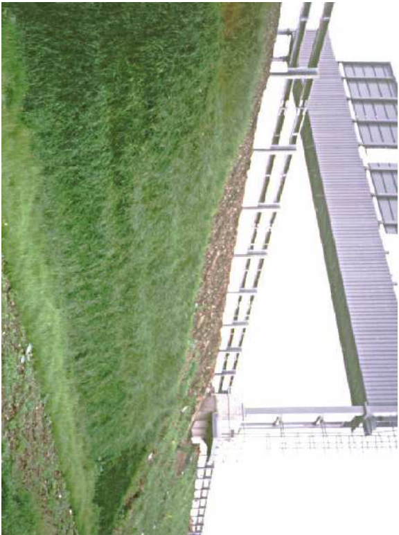
Typical TensarTech GreenSlope Facing.
