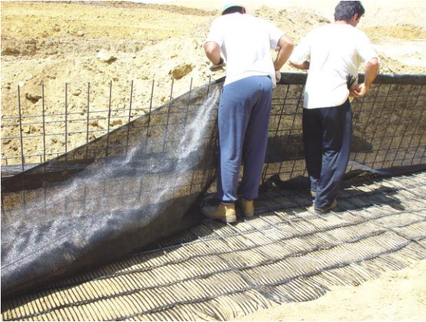
Face liner is rolled out and fixed to the inside of the facing units
