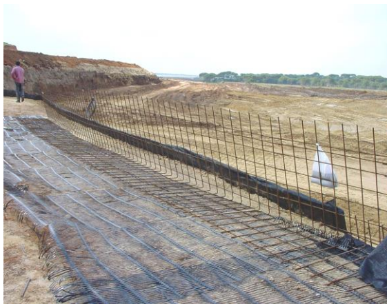
Steel facing units and uniaxial geogrids located in position
