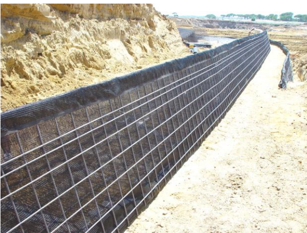
GreenSlope facing units installed and ready for commencement of filling process
