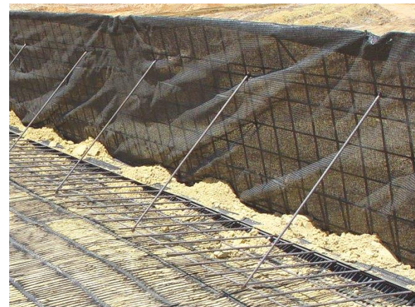
Steel brace bars fixed in to position to maintain the 70° face angle for the long-term
