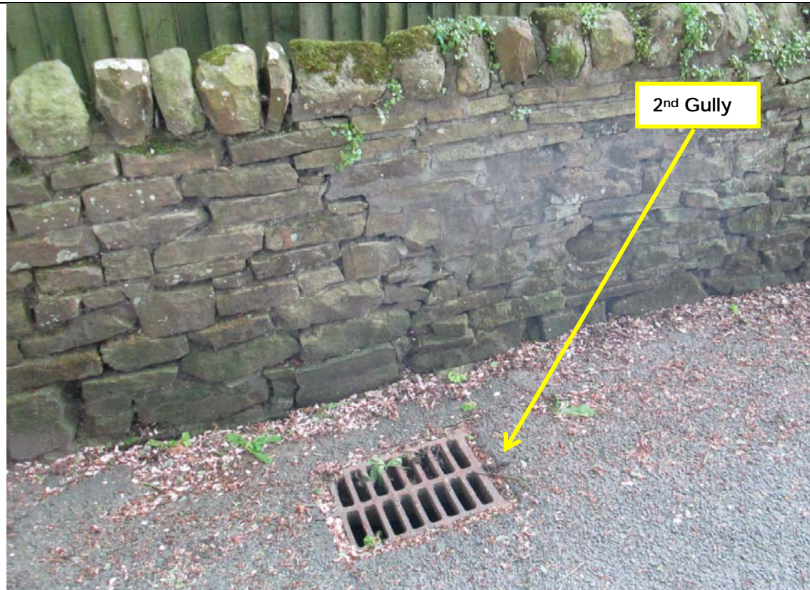
Figure 6.3: Second Downstream Overflow Gully
