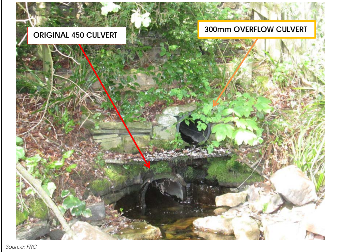
Figure 4.5: Culverts Entering the Site from Whins Lane
