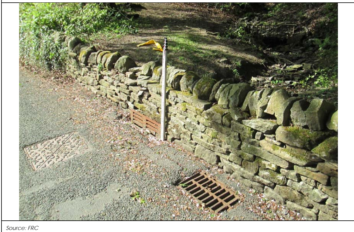
Figure 4.6: Gully discharging into 300mm Overflow Culvert on Whins Lane
