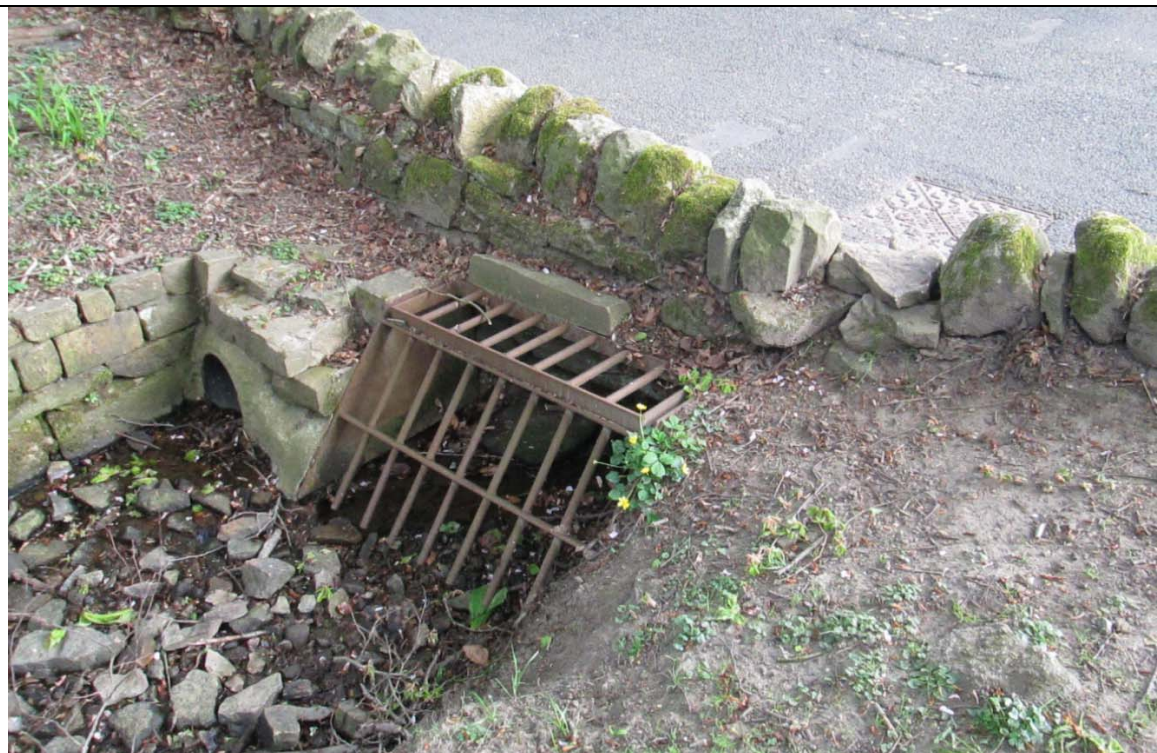
Figure 4.4: Head of Culvert Under Whins Lane
