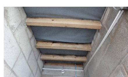
Figure 6: external WC - internal view
