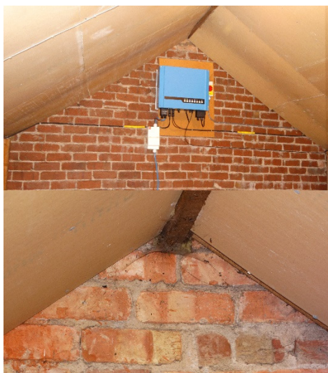
Figure 4: south-east gable end wall
