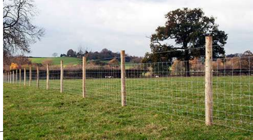
TYPICAL 1200MM HIGH STOCKPROOF FENCE DETAIL
